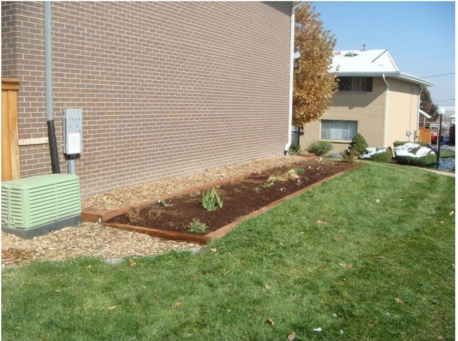
Before renovations, Cherry Creek 3 maintained landscaping from the 1960s. Don Ireland
