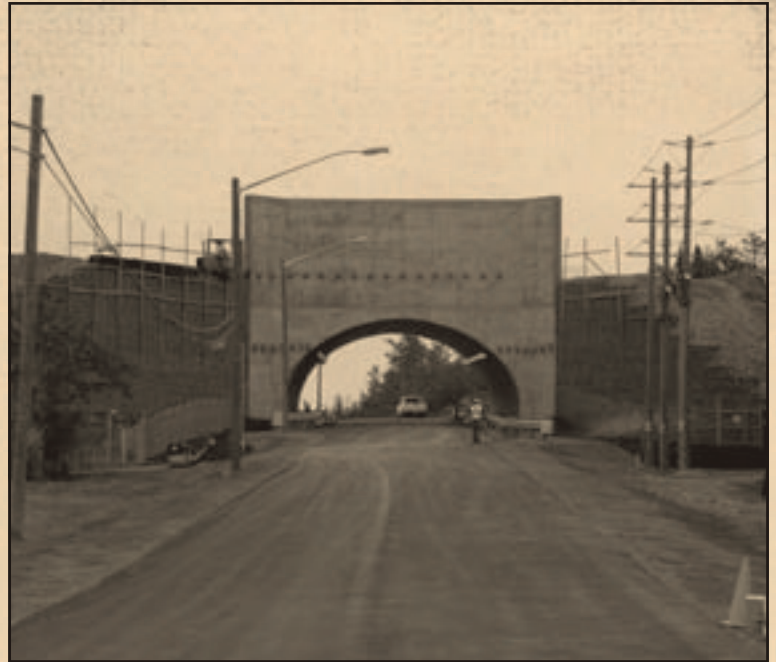
Vipond Road overpass
