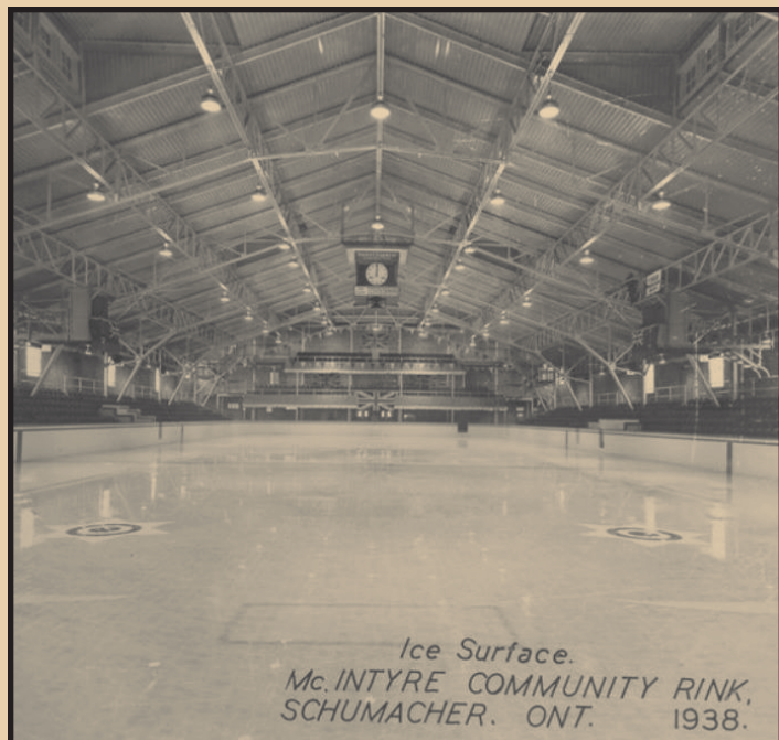
Above: The first page of the McIntyre Community Building Official Opening programme from December 1938 courtesy of Jane Vettor. Below: The newly completed McIntyre arena ice surface. Photo courtesy of Richard Lamoureux.
