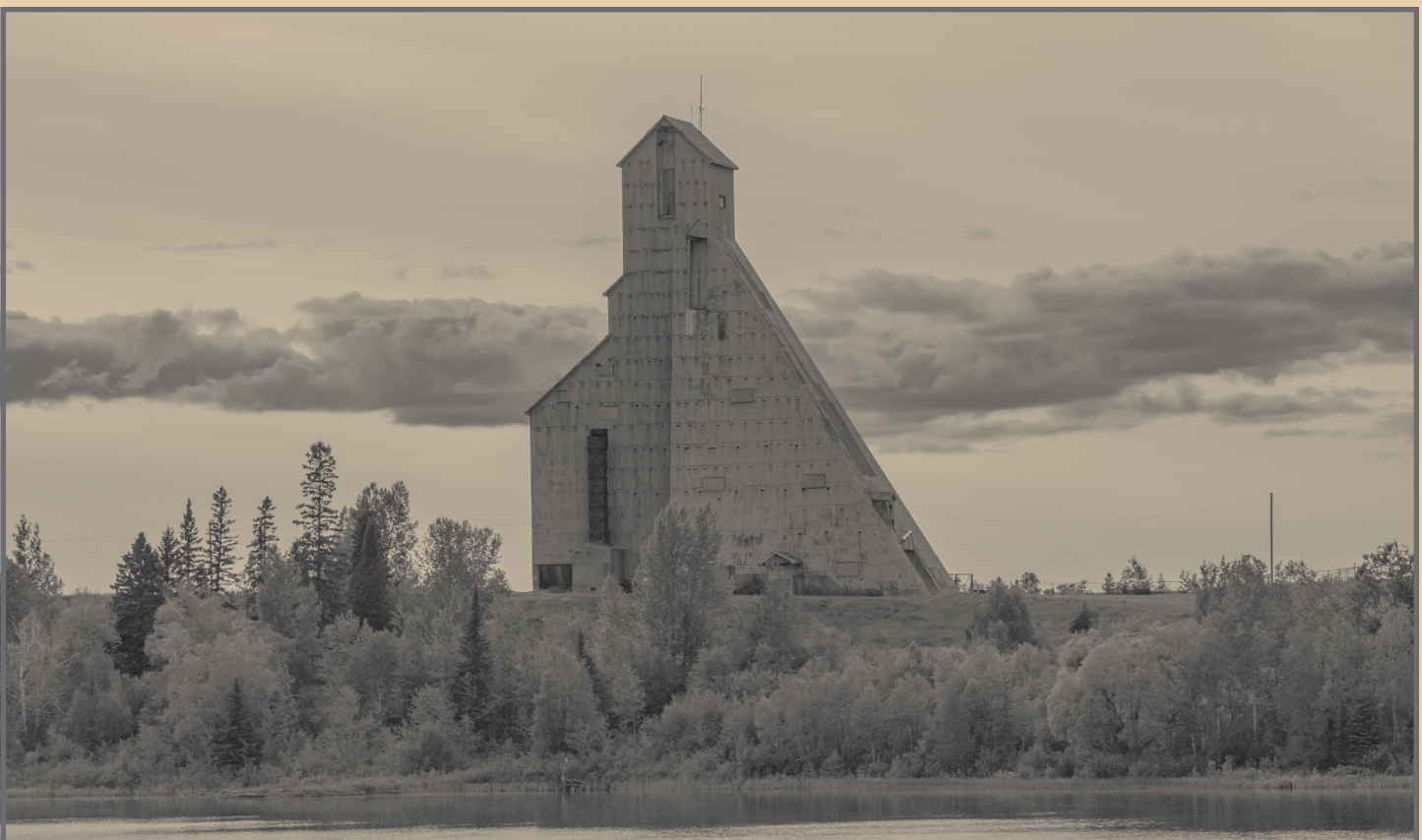
The McIntyre Headframe, which overlooks Pearl Lake in Schumacher, is in need of significant maintenance. (Photo by Lisa Romanowski.)
