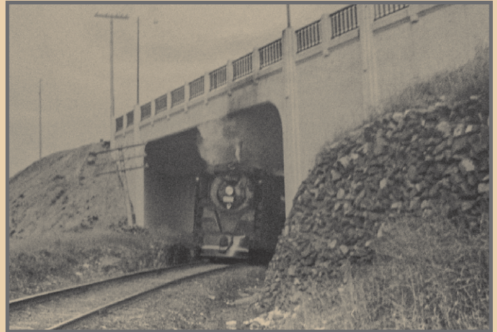
Above: A train passing through the Carium Road Underpass, east of Schumacher. It was constructed in 1939. (Photo courtesy of Norm Moore via Ted Vail.)
