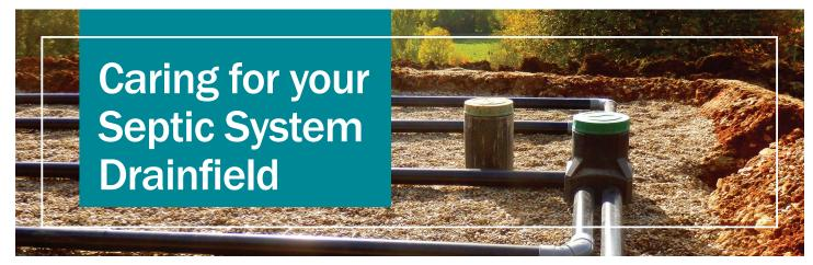
The drainfield includes a network of buried pipes as well as the soil beneath those pipes. Partially treated wastewater from your septic tank is evenly distributed into a network of pipes underneath the drainfield where it is slowly released into the surrounding soil. Natural filtration and microorganisms in the soil remove any remaining harmful particles in the wastewater. The treated and cleansed wastewater then passes into the groundwater and returns to the water cycle.
