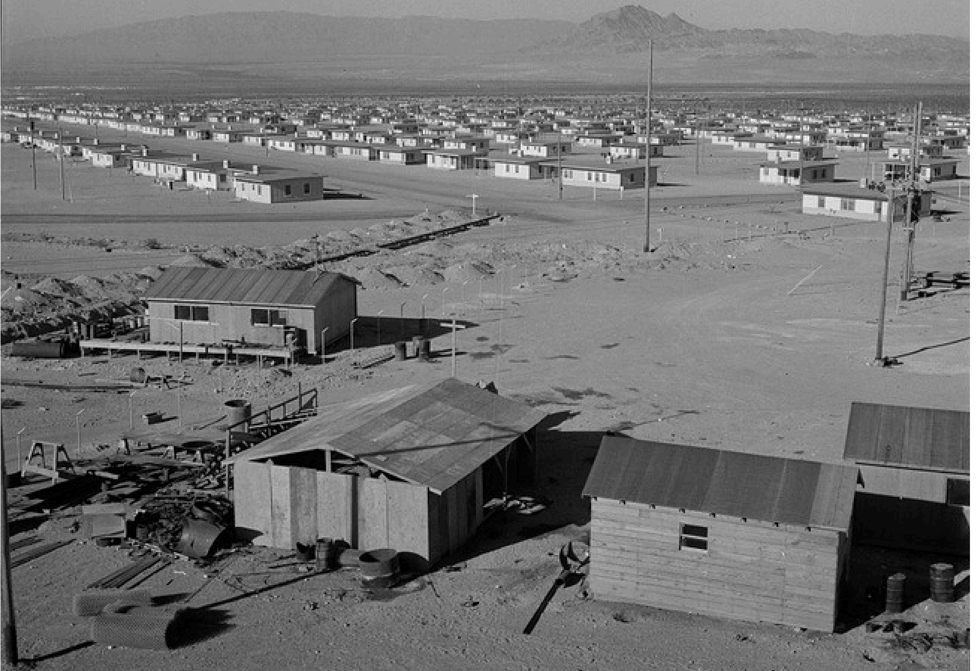
Wartime housing under construction near Basic Magnesium Incorporated, February 1943. Henderson began not as a suburb, but as a federal industrial project built to meet the demands of World War II. Photo by Fritz Henle, Office of War Information. Library of Congress. Public domain.
