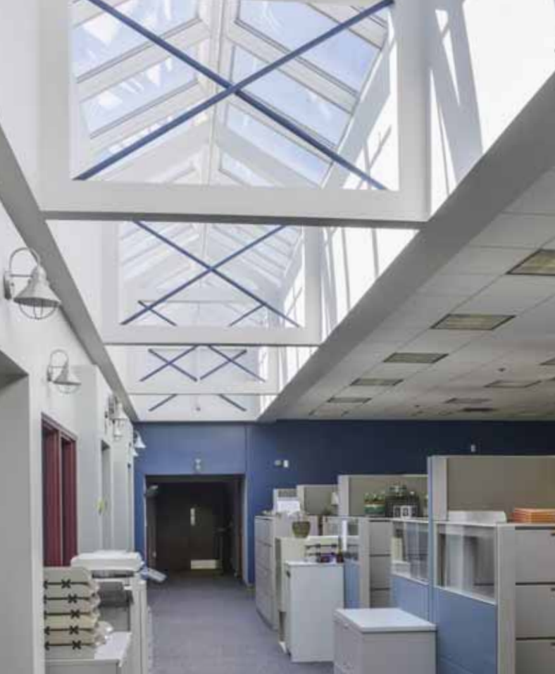
Two VMS Ridgelights replaced two failing translucent panel systems to transform the US Ironworks Facility in Ohio.
