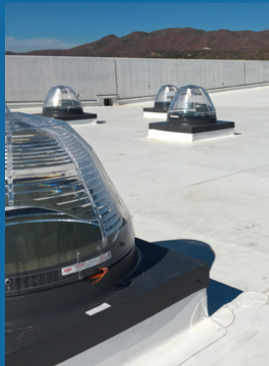
22" kit includes outer dome and VELUX SunCurve
