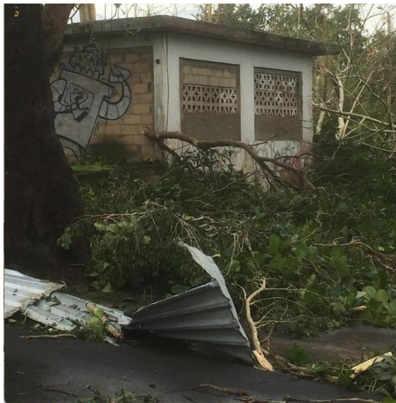
Figure 4: @shittyrobots post from September 23, 2017
