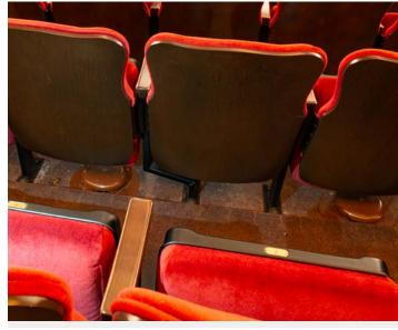
Cantilevered Center Standards (to accommodate building mechanicals)
