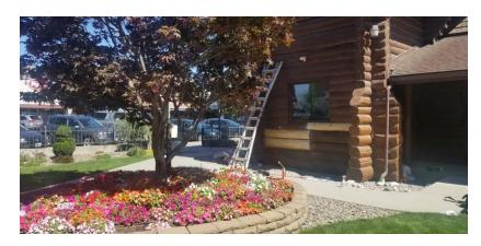
Rimmer and Roeter Construction are onsite at the church this week to complete some much needed log repair. Over time, some of the church logs have cracked and split. Crews are busy replacing, caulking, and sealing them.
