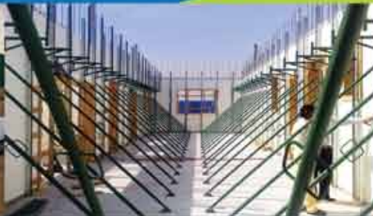
STEP 3 | Prop the walls
