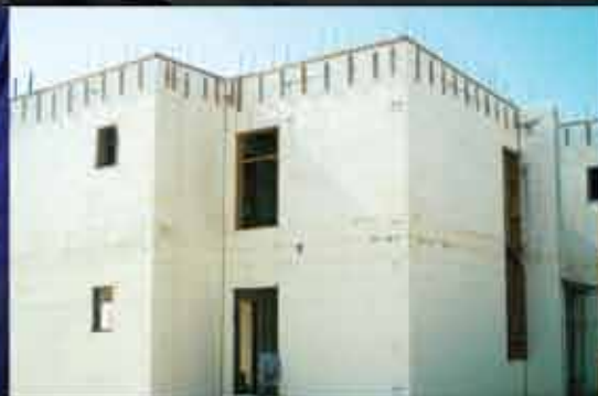
STEP 5 | Core and shell complete
