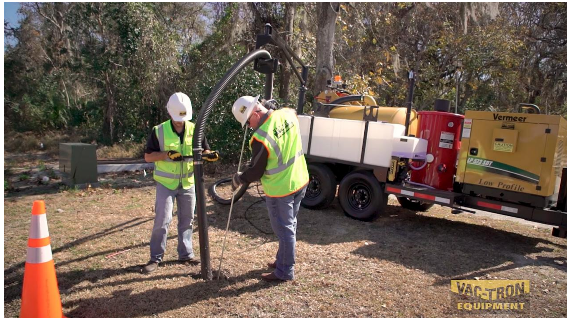
Vac-Tron Vacuum Soil Extraction for Potholing.
