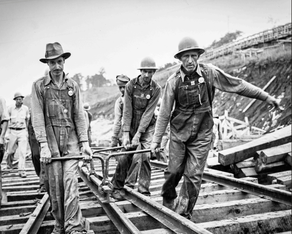
Arthur Rothstein, Laying Track at TVA's Douglas Dam Site. Sevier County, Tennessee, 1942.
