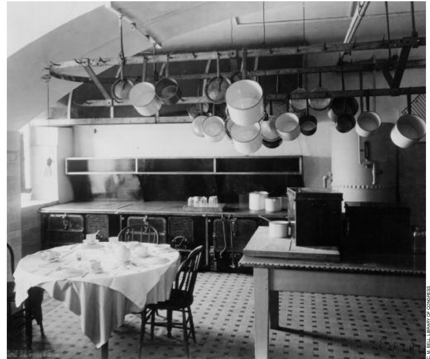
A view of the kitchen in 1901. The large kitchen was used for main events and more formal entertaining. The round table at left is set for a staff meal. The presence of electricity, introduced to the White House in 1891, can be seen by the surface-mounted electrical wiring placed along the ceiling. Single light bulbs hang from the ceiling to illuminate the room; one appears over the round table.
