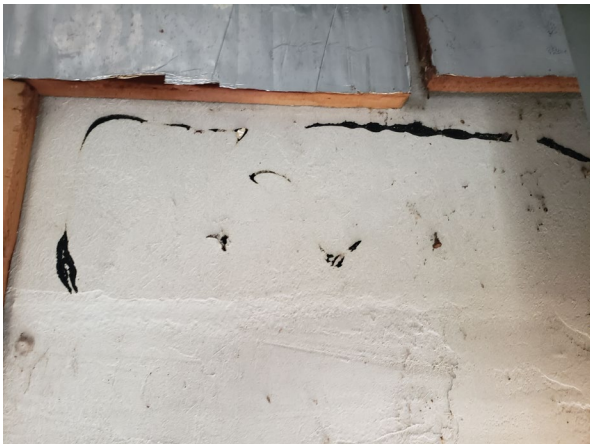
Photograph 9 – 029-01 Foam Insulation Adhesive
