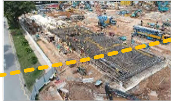
Construction of Fab 1 Starts
