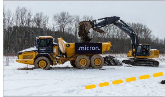
Tree Clearing & Site Prep
