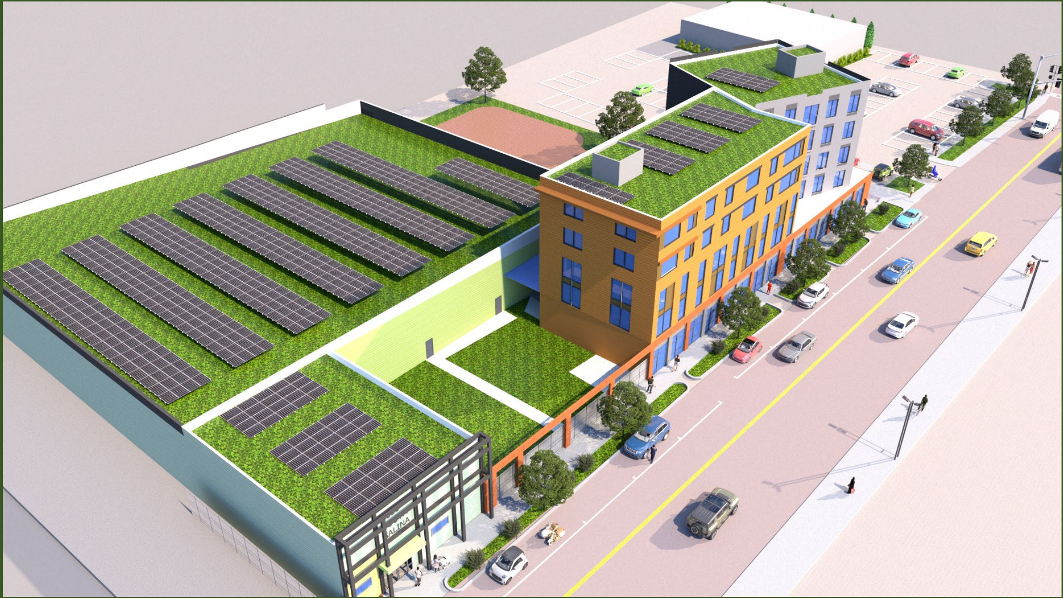
Net Zero – Solar power generation of approximately ½ a megawatt
