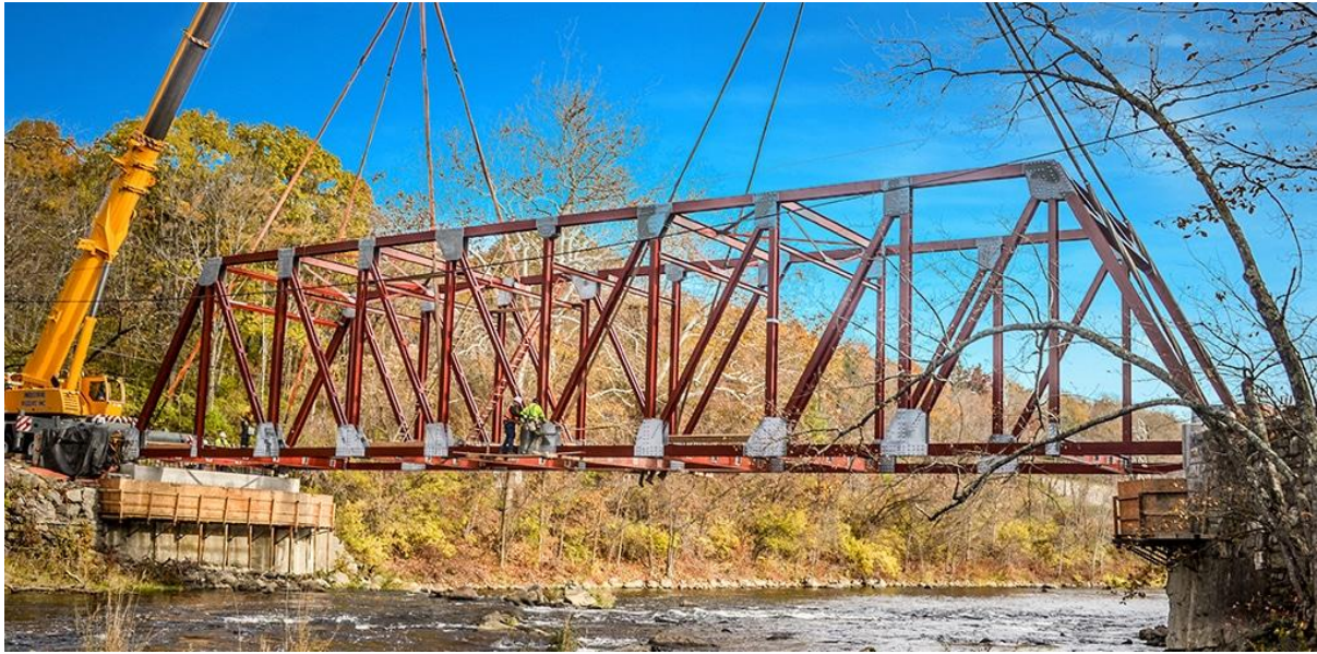
Figure 4 Lifting a truss bridge in its place
