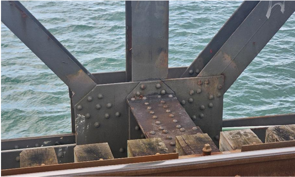
Figure 6 Matapihi Rail Bridge Beam Connection
