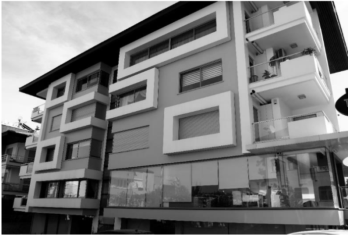
Figure 5. Nursel Kaymakçı Apartment South Facade.
