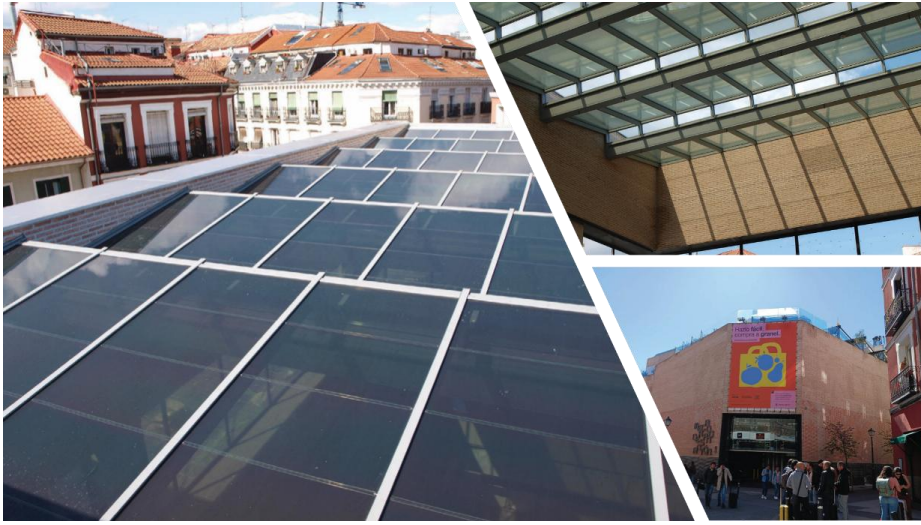
Figure 5. BIPV skylight system implemented in the San Antón Market retrofit project: exterior view of the building from the pedestrian scale (Photograph: Nuria Martín Chivelet, CEMAT) and interior view of the semi-transparent BIPV skylight system (Photograph: Onyx Solar).
