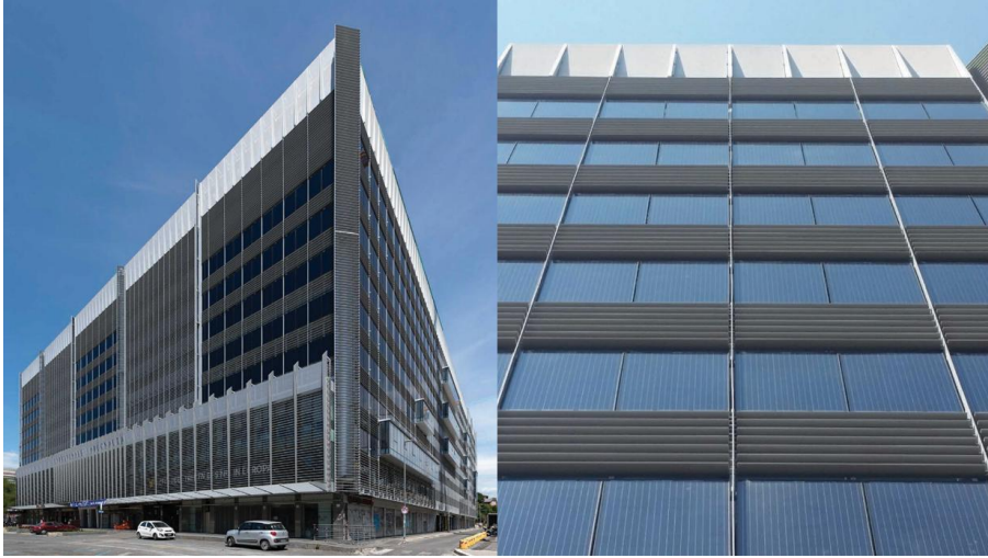
Figure 7. Pre- and post-renovation views and façade detail of the BIPV rainscreen façade system applied in the Palazzo Argonauta project (Photographs: DIARC).
