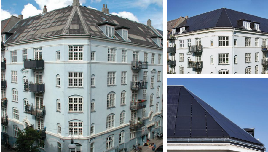
Figure 3. BIPV roof application in the Andreas Bjørns St.1 retrofit project: building views before and after renovation, and roof detail. Credits: Dorte Krogh.
