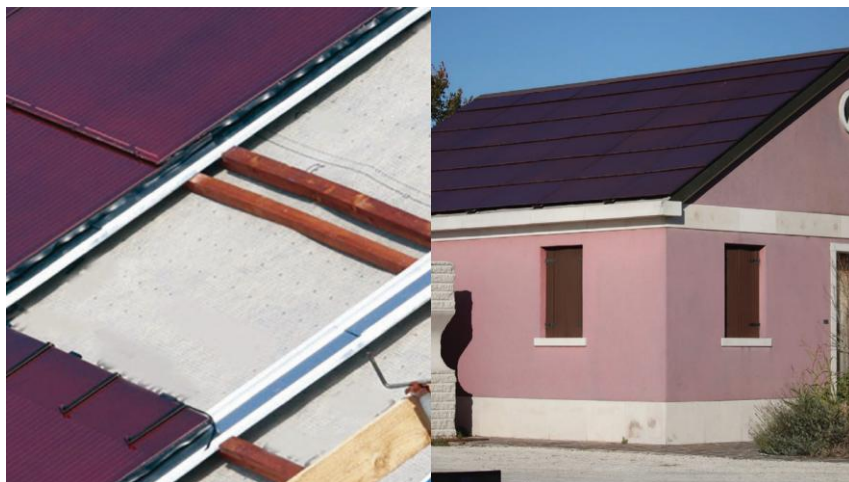
Figure 4. Architectural integration and detail views of the terracotta-coloured BIPV roof modules applied in the Certosa Island Urban Park retrofit project. Credits: GruppoSTG.
