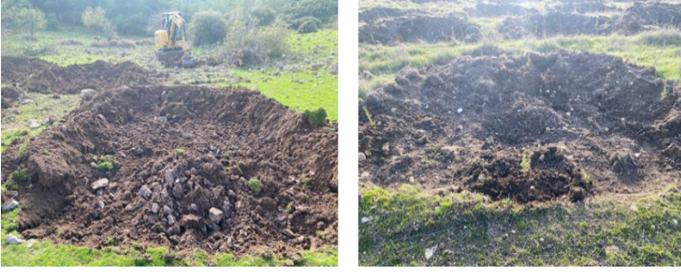
Figure 9: Crescent-shaped bunds (6×6 m) implemented in İzmir, Türkiye (Photo: Muhammed Ali AYDIN).
