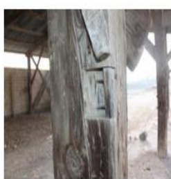
Figure 16. Evidence for the shed restitution: (a) support traces on the bracing of axis A; (b) secondary-beam traces on columns 2/A and 2/I; (c) dovetail detail; (d) remains of façade timber, nail traces, holes in columns and iron profile.
