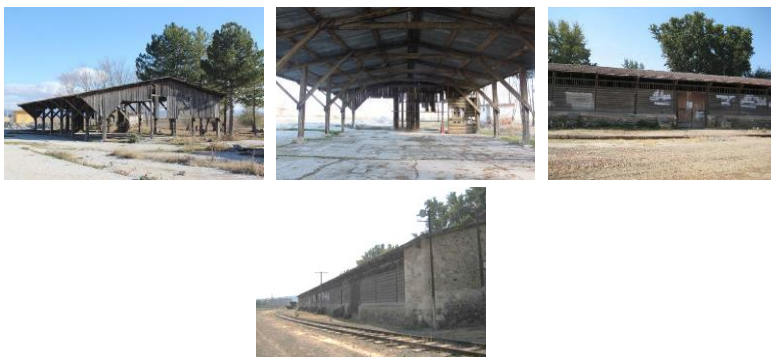
Figure 17. Comparison of the shed buildings: (a) west façade of the Çardak shed building and front façade of the Evciler shed; (b) east façade of the Çardak shed building and rear façade of the Evciler shed building; (c) remains of timber eaves cladding and nail marks on the Çardak shed building; (d) façade timbers and railings of the Evciler and Sarayköy shed buildings.
