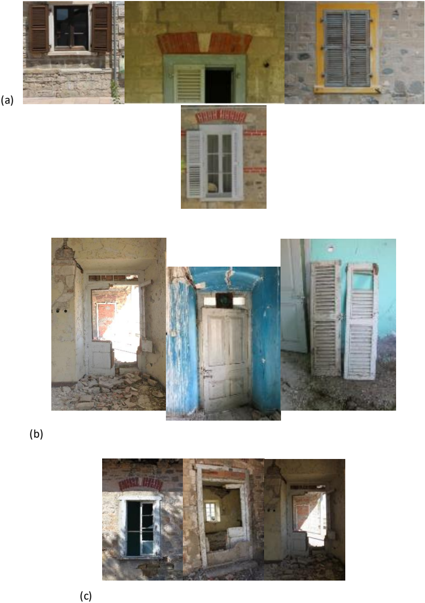
Figure 13. Comparative details: (a) shutter systems of stations on the line; (b) Evciler double-leaf door, hinge and louvre details; (c) door and window types of Evciler Station Building.
