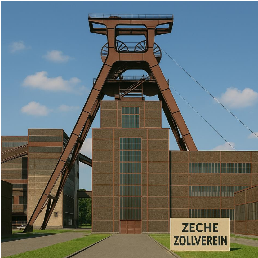
Figure 15 Zollverein Coal Mine Industrial Complex in Essen
