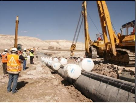
Settling down the pipe, floats is fixed on the pipe (from BOTAŞ archive, March 2004)
