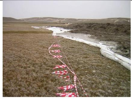
Turf protection using geotextile during subsoil stockpiling (March 2004)
