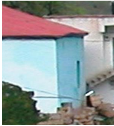
Figures 7,8 Southern Façade (Sedes, 2014)
