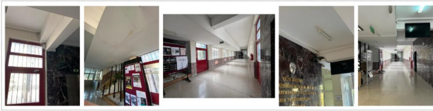
Figure 2. Images of the Corridor's Current Condition
