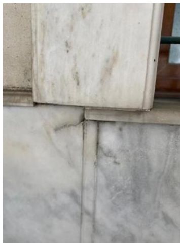
Figure 1. Example of cracks observed on a building facade (Original, 2025)
