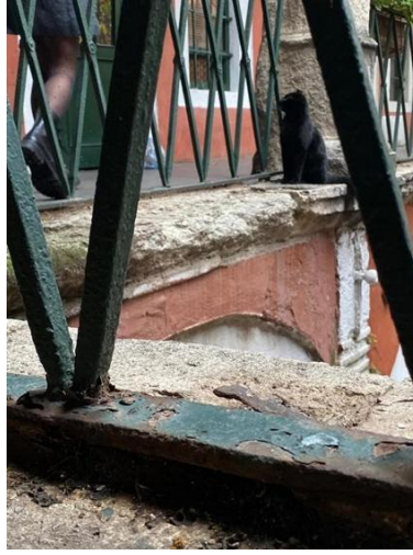
Figure 4 Chemical deterioration and corrosion observed on Zincirli Han (Original, 2025)
