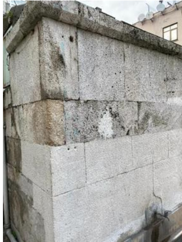
Figure 2 Erosion observed on Çandarlızade Atik İbrahim Pasha Mosque (Original, 2025)
