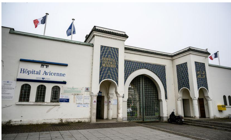
Figure : Entrance to Ibn Sina Hospital in Bobigny (Seine-Saint Denis), France Source: Taken from the Assistance Publique – Hôpitaux de Paris website
