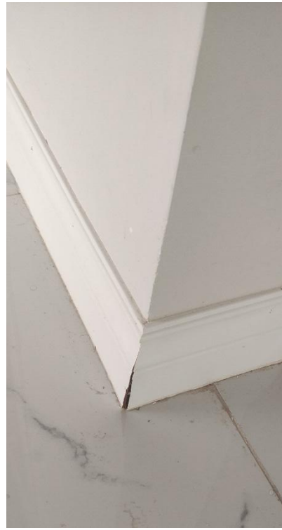
Figure 25: Radiator pipes aligned very close to the wall surfaces. Figure 26: Wear seen at corner joints of wooden baseboards.
