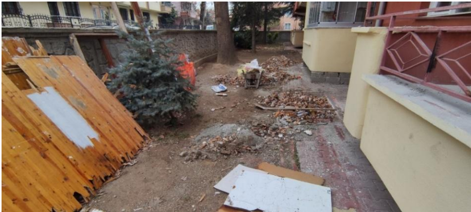
Figure 19: Wooden parquet flooring that was broken and removed from the house.
