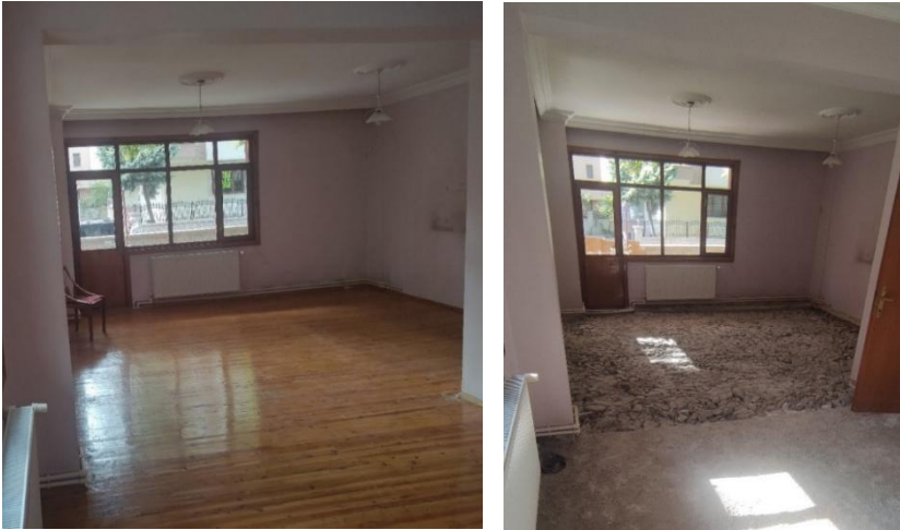
Picture 4: Living room wooden flooring to be removed
