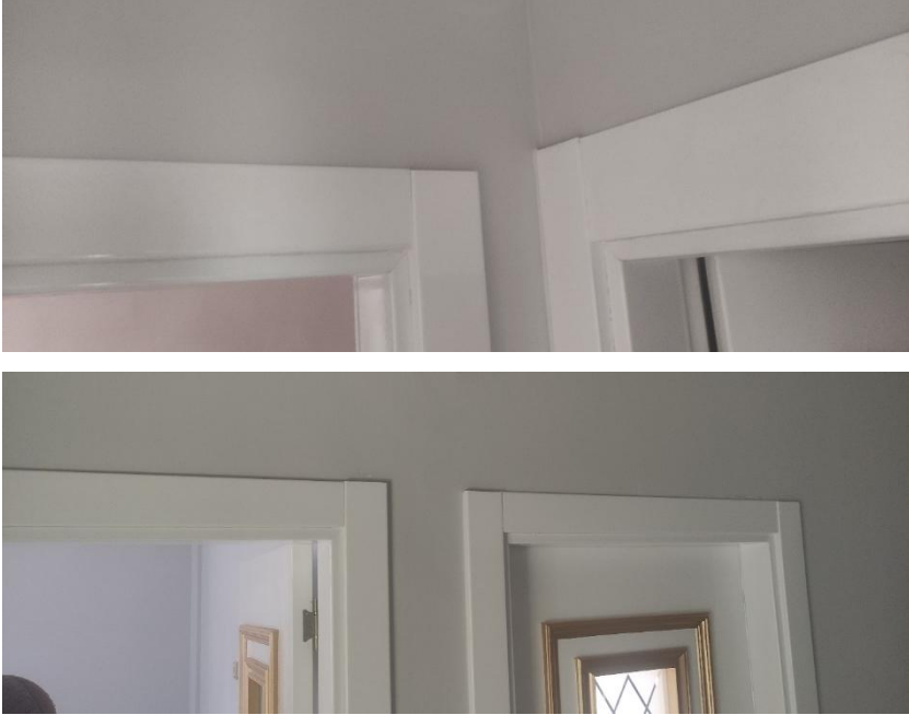
Figure 24: Alignment problem at the top of the door
