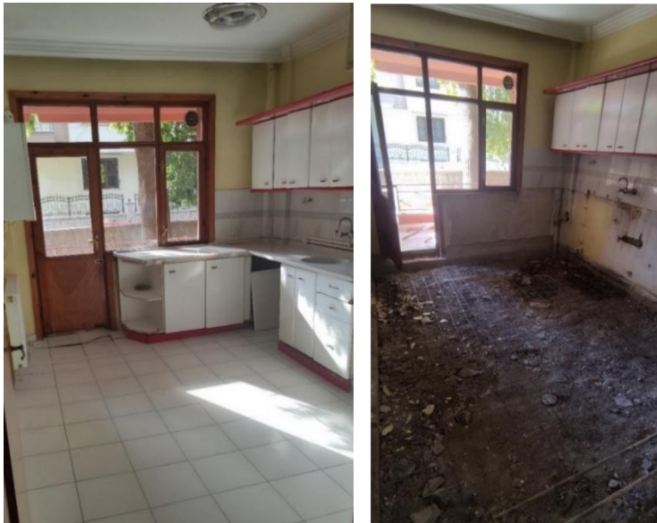
Figure 5: Kitchen Ceramic Flooring to be Removed
