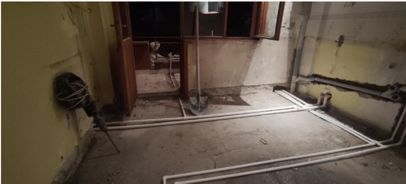
Figure 7: Renovated and underground water and heating pipes.
