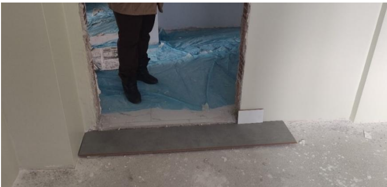
Figure 14: Ground level discrepancy in the place where laminate flooring will be installed
