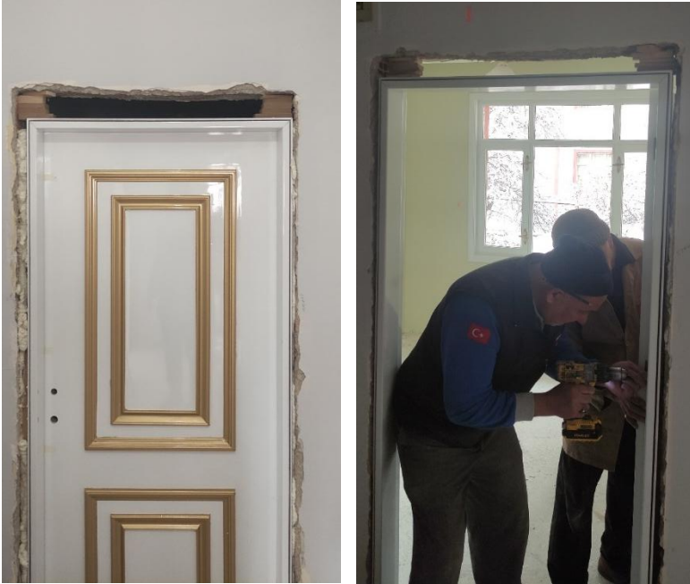
Figure 15: Lacquer coating door installation
