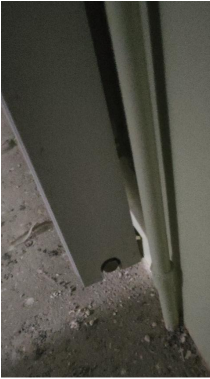
Figure 25: Radiator pipes aligned very close to the wall surfaces. Figure 26: Wear seen at corner joints of wooden baseboards.
