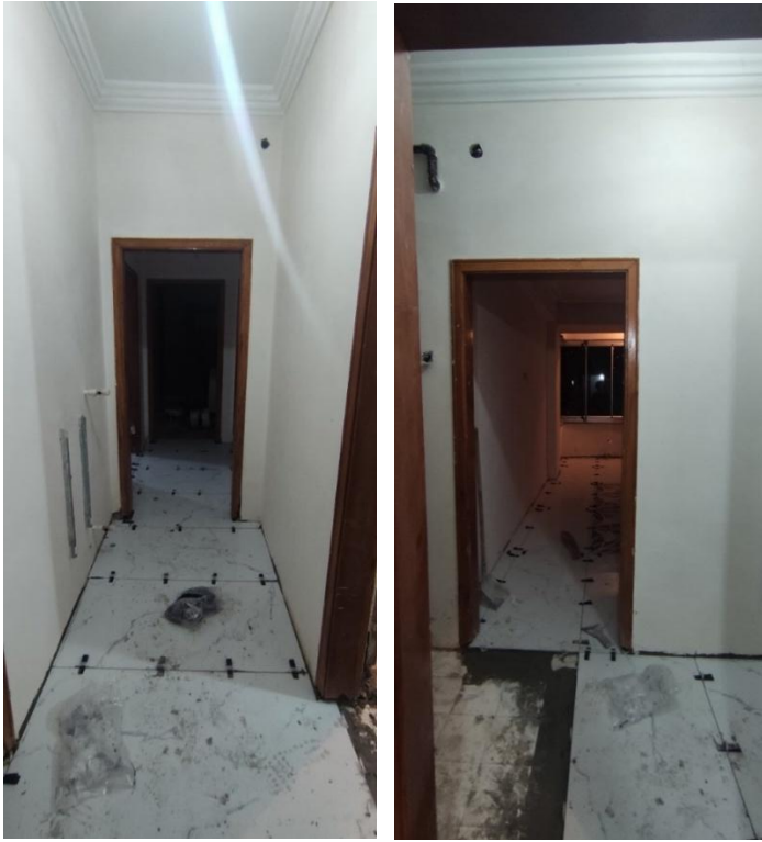
Figure 13: Tile flooring application
