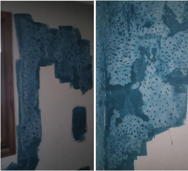
Figure 21: Primer application before plastering to improve integration.
