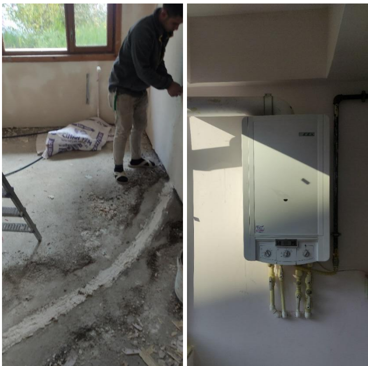
Figure 12: Electric lines drawn from the floor and wall
