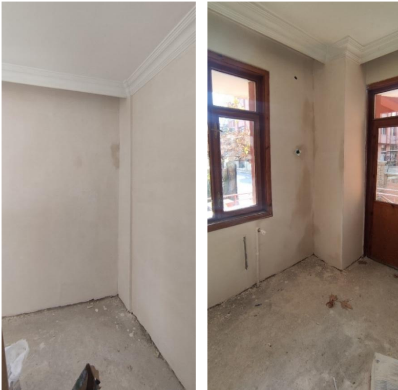
Figure 11: Plastering and painting applications on the walls.
