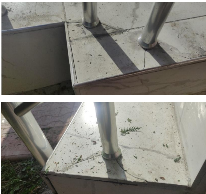
Figure 29: Tiles damaged when opening the railing connection points
