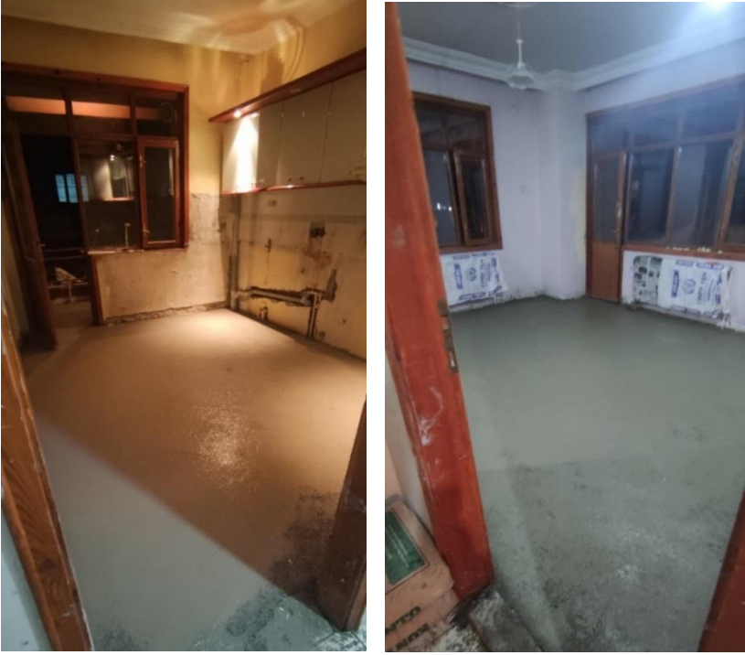
Figure 8: Floor leveling applied by pouring screed concrete
