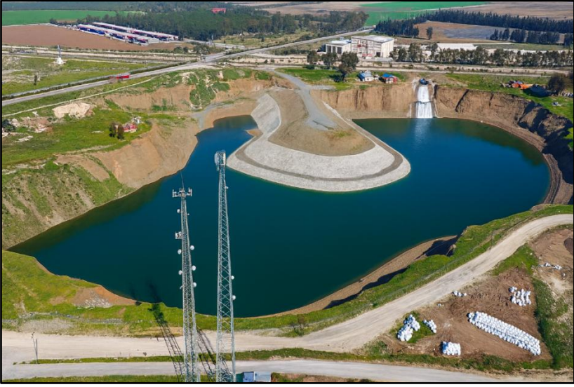
Figure 2. Serinyol underground dam (Hatay)(Soz Newspaper, 2022).
