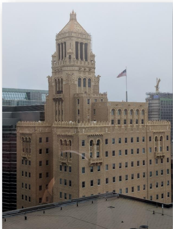
Original Mayo building
