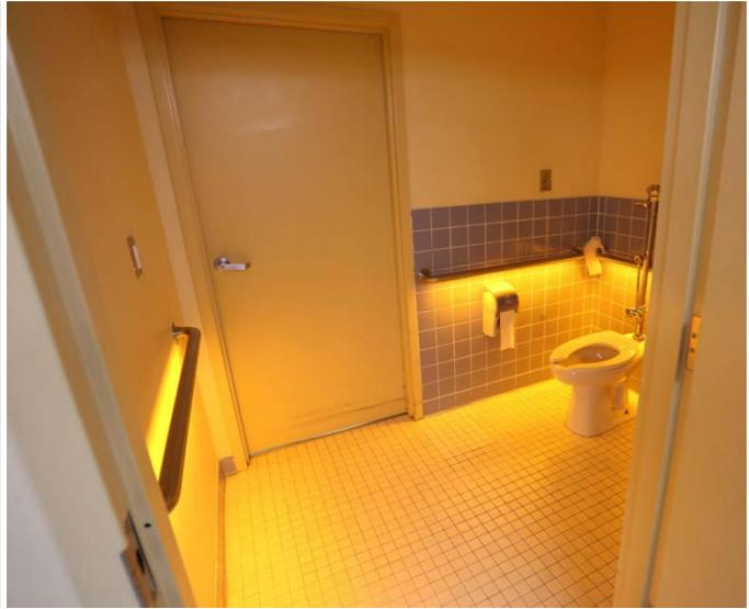
**Figure 14: Nighttime lighting elements that promote good sleep hygiene. Amber rope lights were installed underneath each bed, controlled by motion sensors that would respond at night to someone getting out of bed or to a nurse entering the room (left photo). Amber LED lighting was also integrated into new handrails in the bathrooms, controlled by motion sensors to provide low-level lighting when someone entered the bathroom (right photo).**
