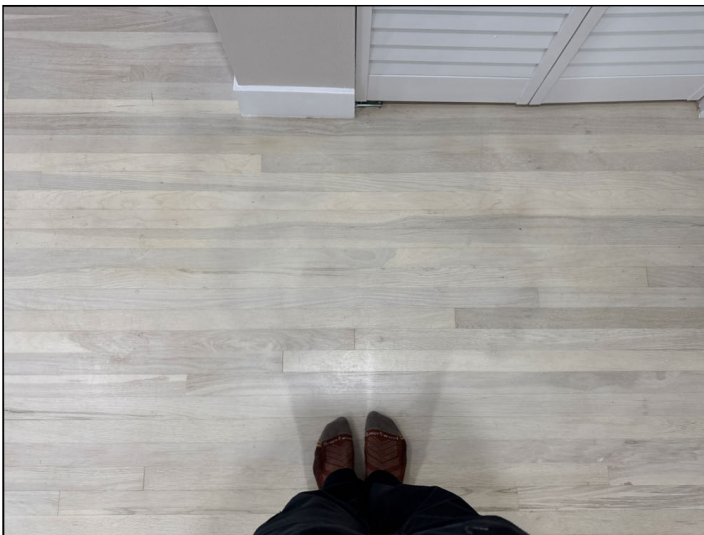
Floor boards are loose and noisy. Repairs are needed.
