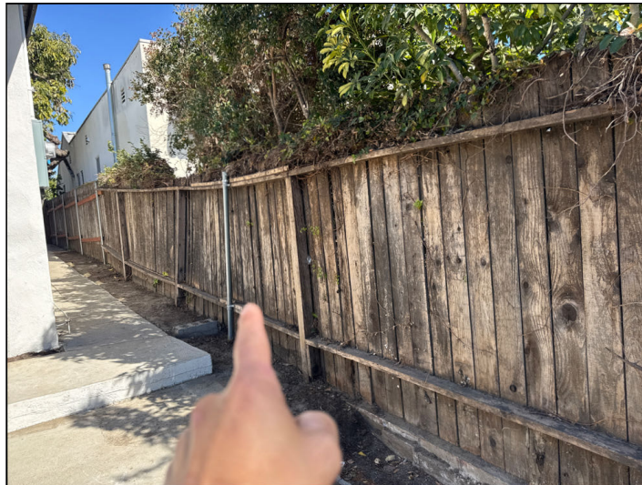
Fence is leaning or falling. Repair or replacement is recommended.
