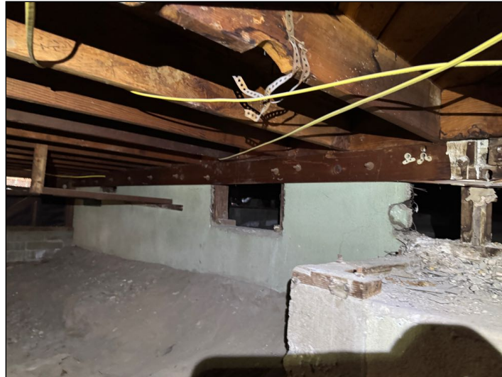
Access panel is not installed. Installation is recommended.
