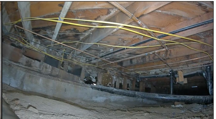
Moisture, rot or termite-like damage noted under the floor joists.
