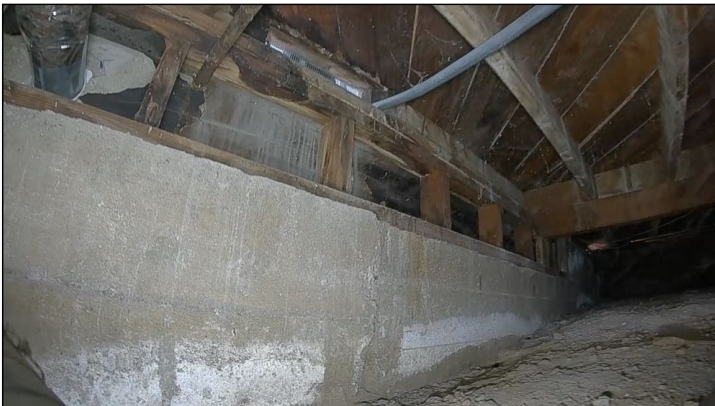
Efflorescence observed on walls indicates the presence of periodic moisture.
