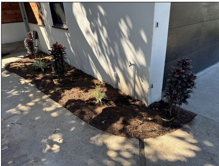
Planter areas near the house do not have a drainage system installed and retain water when it rains. This excess moisture, near the foundation of the house, can cause damage. Installation of a drainage system is recommended.
