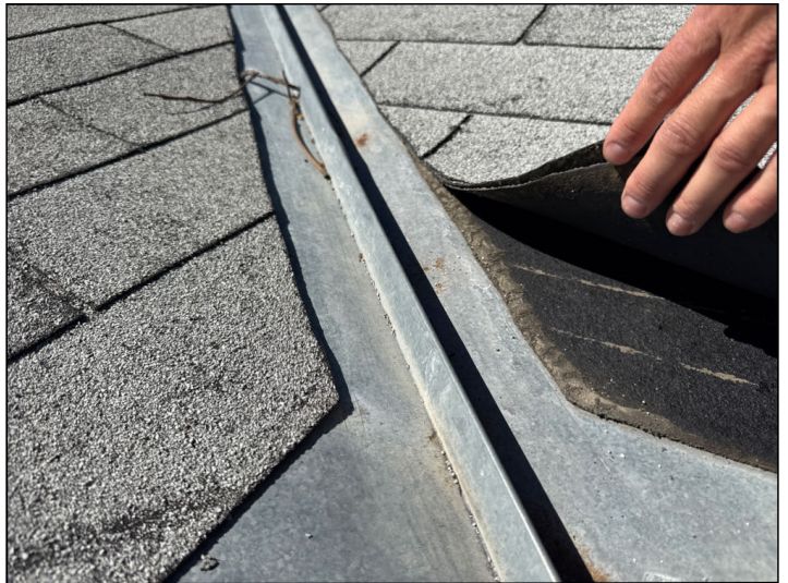
Flashings do not appear to be properly sealed at the valley.
