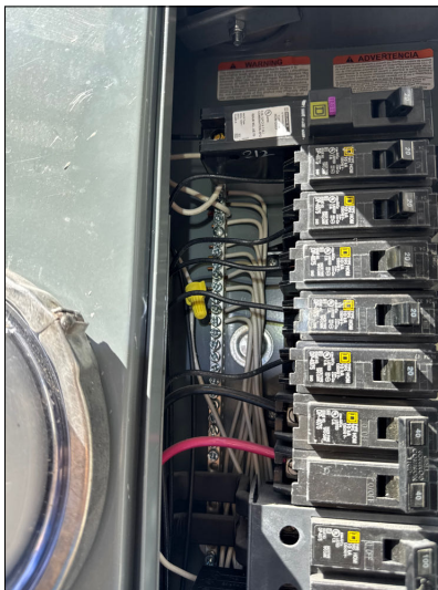
Grounding system is present.
