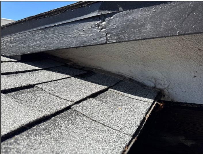
Flashing is not installed at the wall junctions.
