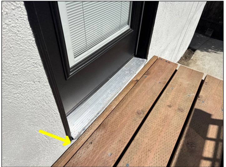
Flashings are not properly sealed at the floor to wall junction and may allow moisture penetration and damage.
