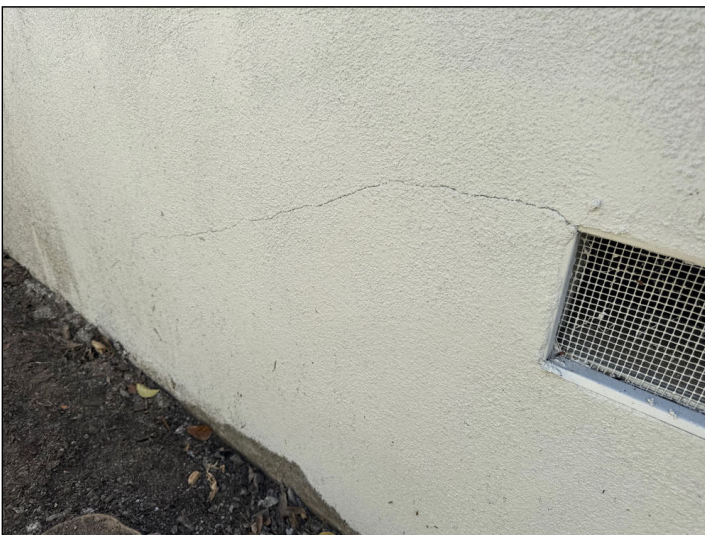
Cracks noted are moderate and may indicate foundation movement due to seismic activity or settlement.
