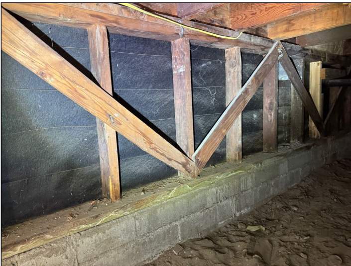
Moisture, rot or termite-like damage noted on the mud sills and or cripple walls.
