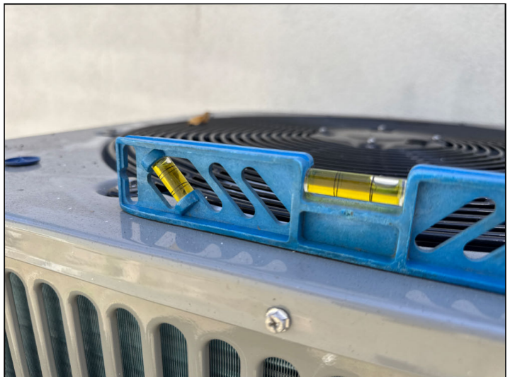
Condenser unit is visibly unlevel and may not allow proper operation of the refrigeration pump. Leveling is recommended.
