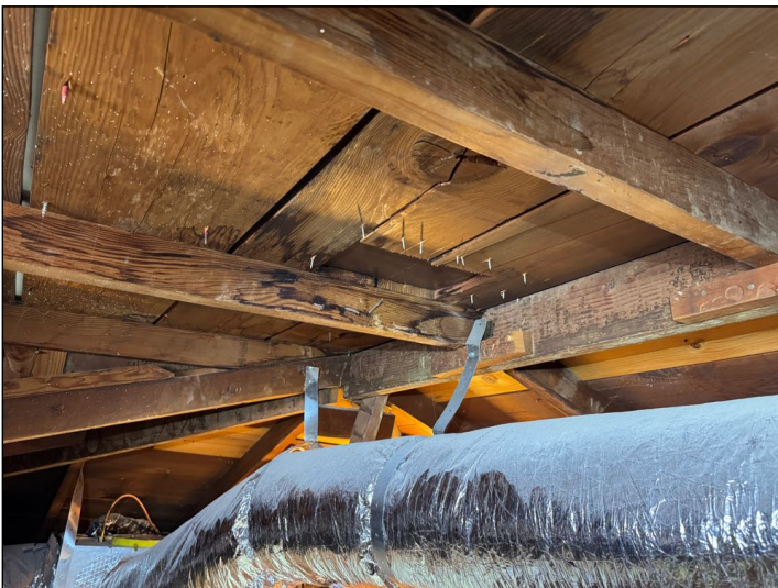
Unable to determine the status of the stains. Active leakage may be present.
