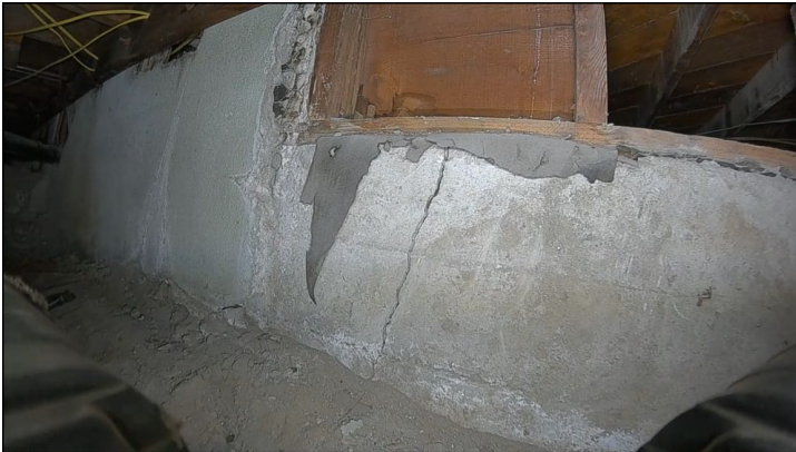
Minor settlement cracks noted on the foundation stem walls at one or more location. Cracks do not appear to be significant at this time.
