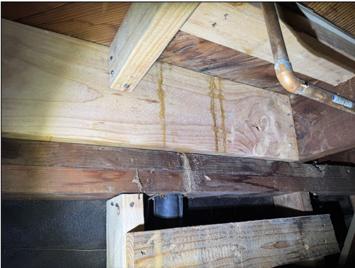
Moisture, rot or termite-like damage noted under the bathroom.
