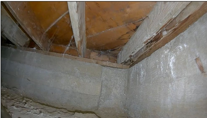
Moisture, rot or termite-like damage noted on the mud sills and or cripple walls.
