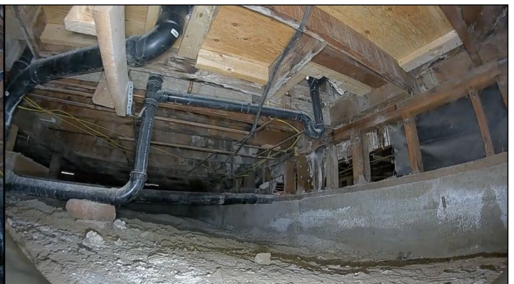
Moisture, rot or termite-like damage noted under the bathroom.
