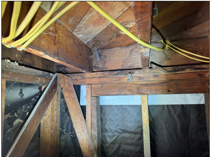
Moisture, rot or termite-like damage noted under the floor joists.
