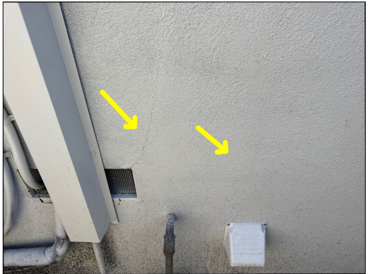
Cracks are typical and not structurally significant.
