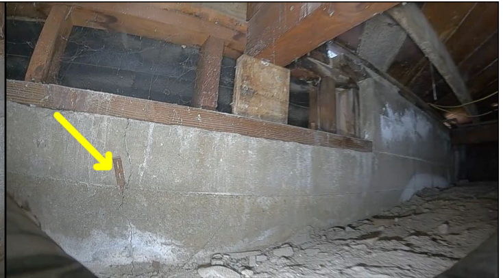
Moderate settlement cracks noted on the foundation stem walls at one or more location. Cracks do not appear to be significant at this time.
