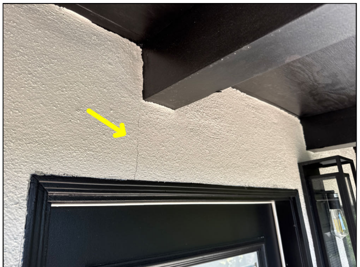
Cracks are typical and not structurally significant.
