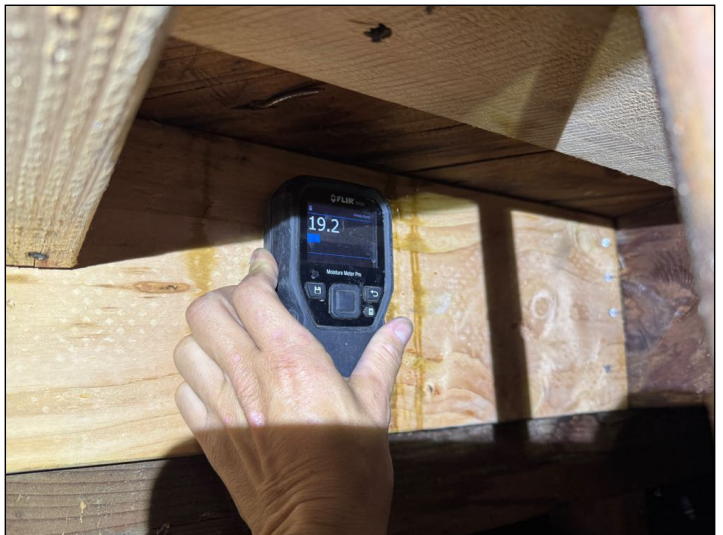
Active moisture intrusion into the building by materials was confirmed at the time of inspection with the use of a moisture meter. Building materials with a moisture content above 20% will allow for mold spores to reproduce. Recommend further evaluation and mold sampling by a qualified contractor prior to the close of your transaction.
