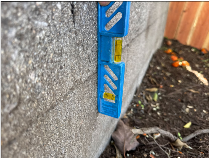
Block wall is leaning or falling. Repair or replacement is recommended.
