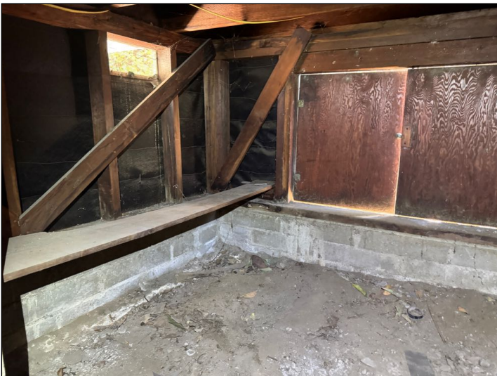
Cripple walls are present, but not braced. Reinforcement is recommended but may not be required.
