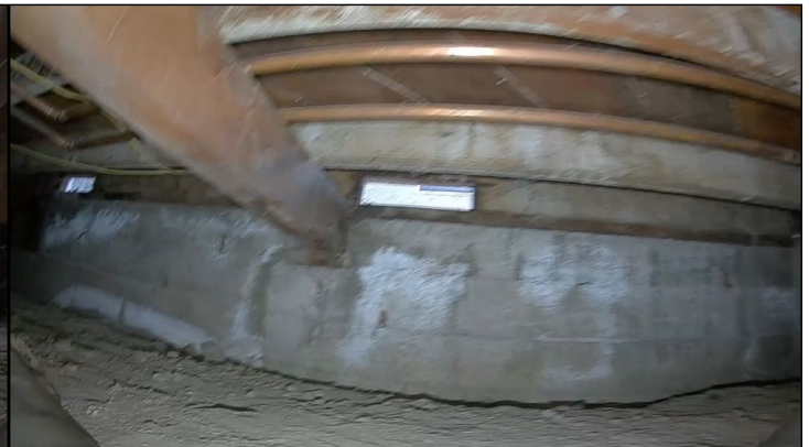
Efflorescence observed on walls indicates the presence of periodic moisture.
