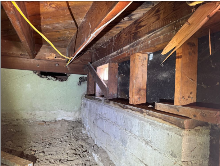
Anchor bolts are installed. Wood frame appears to be bolted to the foundation.
