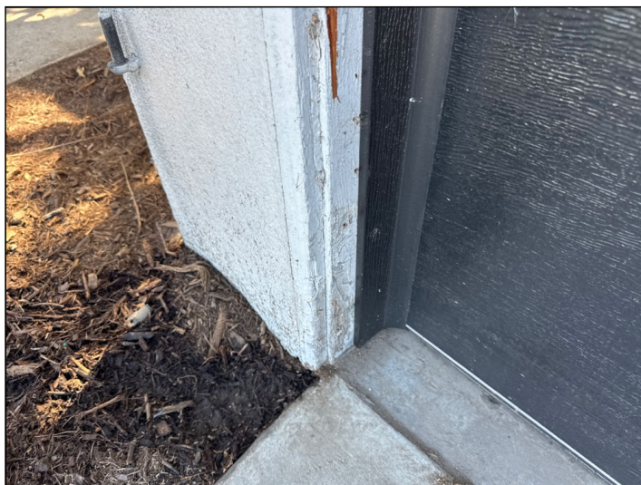
Paint finish is flaking or deteriorated. Repainting is recommended.
