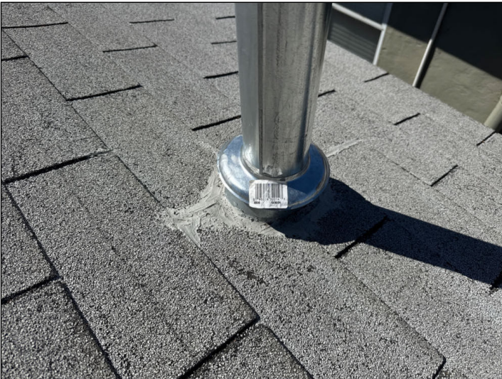
Flashings do not appear to be properly sealed at the vent pipes.
