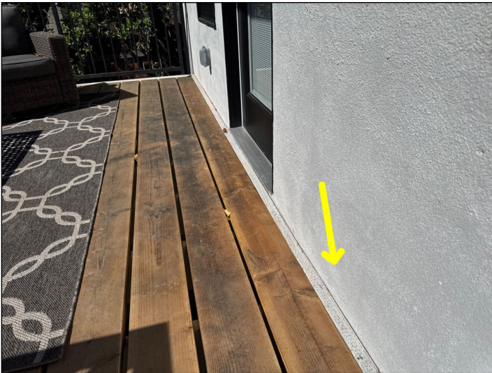
Flashings are not properly sealed at the floor to wall junction and may allow moisture penetration and damage.
