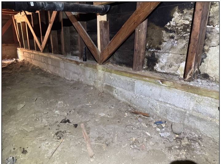
Efflorescence observed on walls indicates the presence of periodic moisture.
