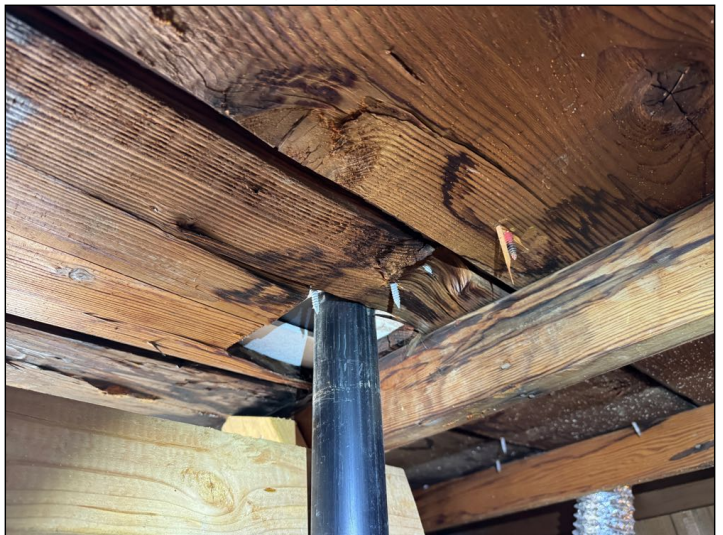
Moisture stains observed at the vent pipes.
