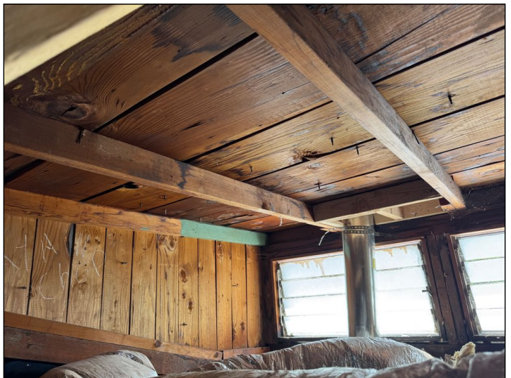
Minor staining was noted on the wood surfaces in the attic, indicating a possible roof leak.
