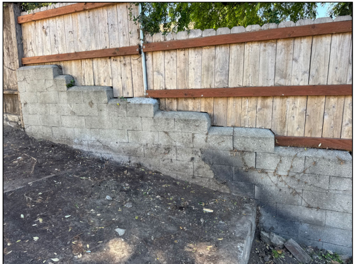
Moderate cracks noted on the block wall.
