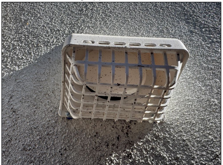
Dryer venting is provided.
