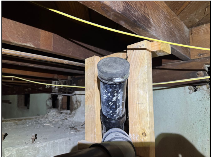
Drain line clean out is not readily accessible. Installation of an extension on the pipe is recommended for easier access for inspection, maintenance and repairs of the sewer lines.
