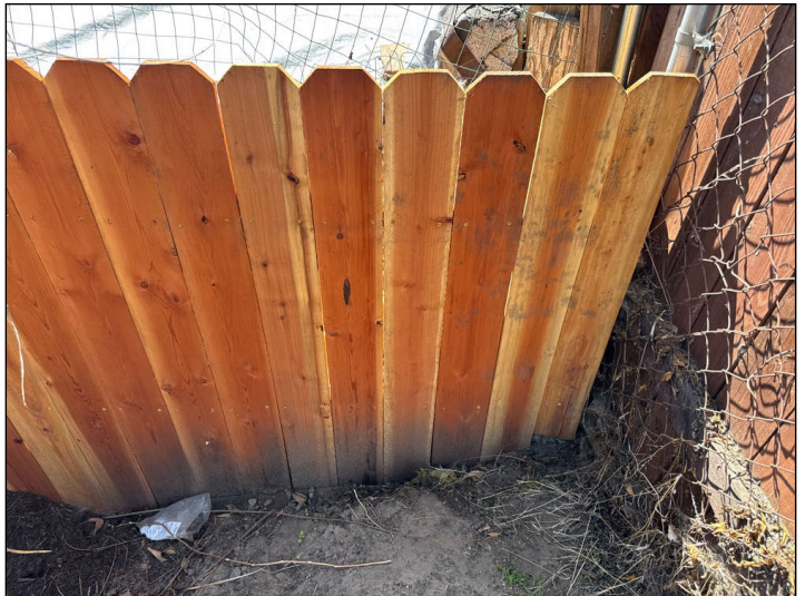
Earth to wood contact observed at the wood fence. A minimum 6 inch separation is recommended between the soil and the bottom of the fence to prevent moisture penetration and damage.
