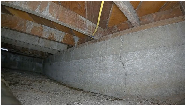
Moderate settlement cracks noted on the foundation stem walls at one or more location. Cracks do not appear to be significant at this time.
