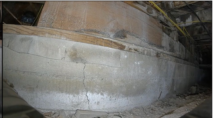
Minor settlement cracks noted on the foundation stem walls at one or more location. Cracks do not appear to be significant at this time.
