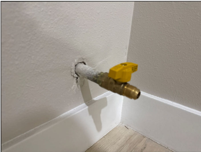
Gas service pipe is provided.
