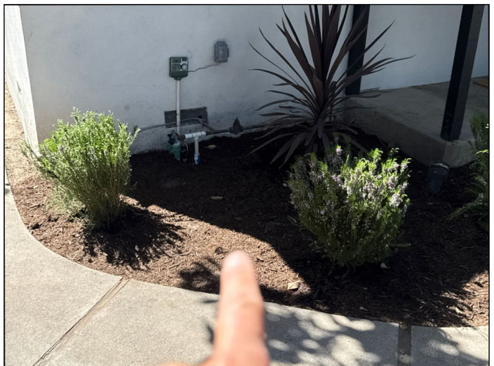
Improper soil slope toward foundation. Slope should fall away from the foundation at a minimum of 1/2 inch per foot and extend at least 10 feet away from the foundation.
