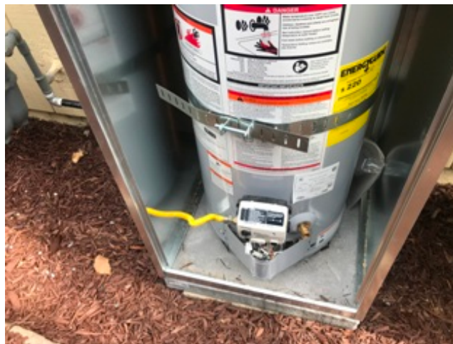
Unsafe Installation of Water Heater Gas Line
