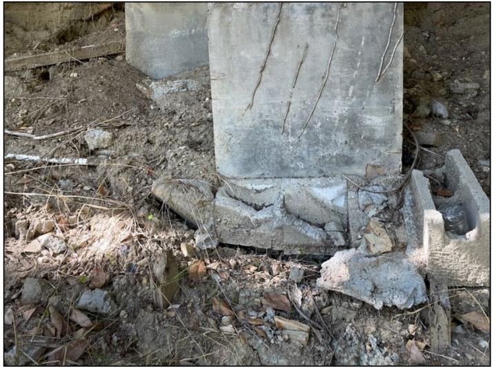
Significant soil erosion under the deck at the supports. Support is visibly leaning.
