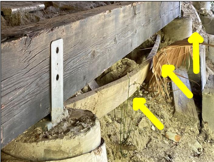
Soil erosion prevention boards collapsed.
