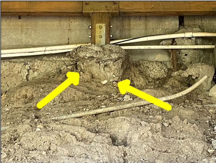
Significant soil erosion under the deck at the supports.
