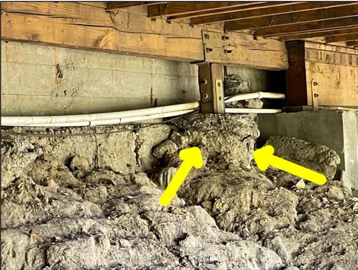
Significant soil erosion under concrete pier supporting the deck
