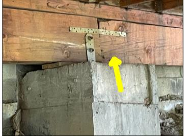
Soil erosion prevention boards collapsed.
