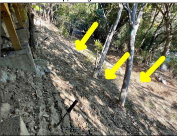
Inadequate hillside coverage. Evidence of significant soil erosion
