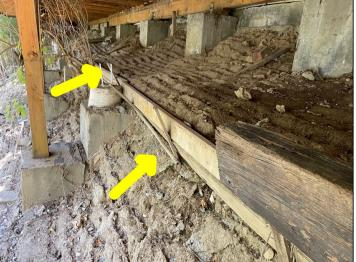
Improper 6 ft cantilever
