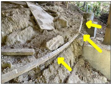
Soil erosion prevention boards collapsed.
