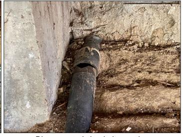
Inadequate connection to concrete support
