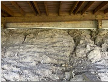
Significant soil erosion under the deck at the supports.
