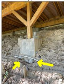
Significant soil erosion under the deck at the supports.
