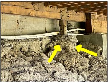
Significant soil erosion under concrete pier supporting the deck
