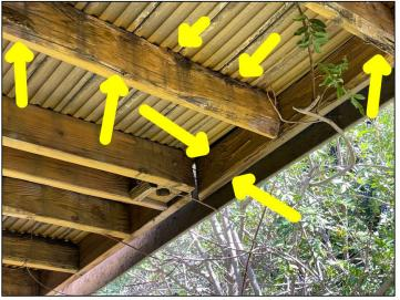
Rot damage. Rim joist is falling off.
