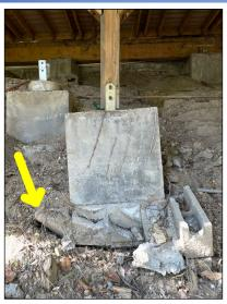
Significant soil erosion under the deck at the supports. Support is visibly leaning.
