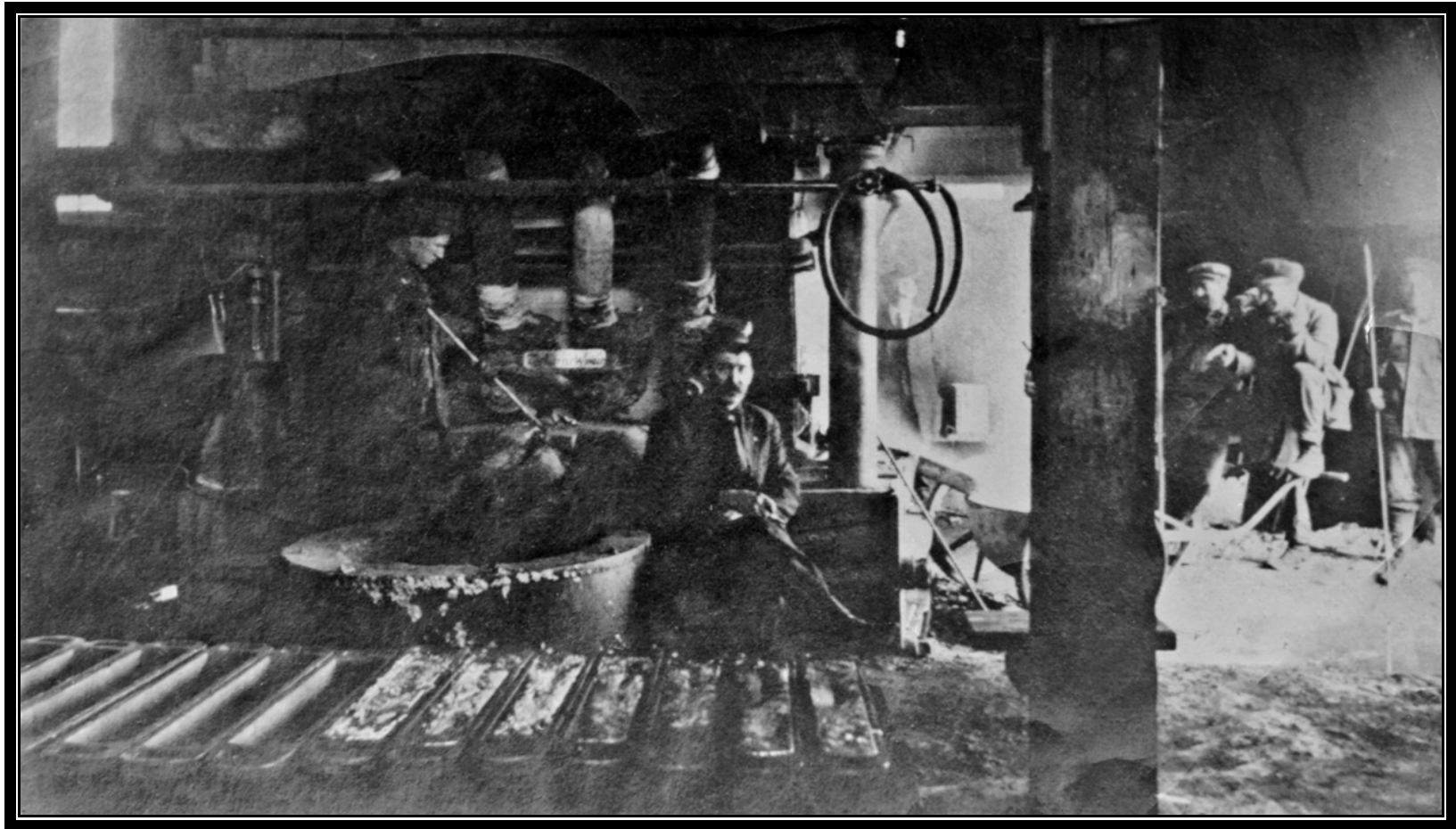
Figure 8. Casting bullion bars in the Clayton smelter, c. 1912. Photograph used courtesy of Clayton Area Historical Association ( www.claytonidaho.org ).
