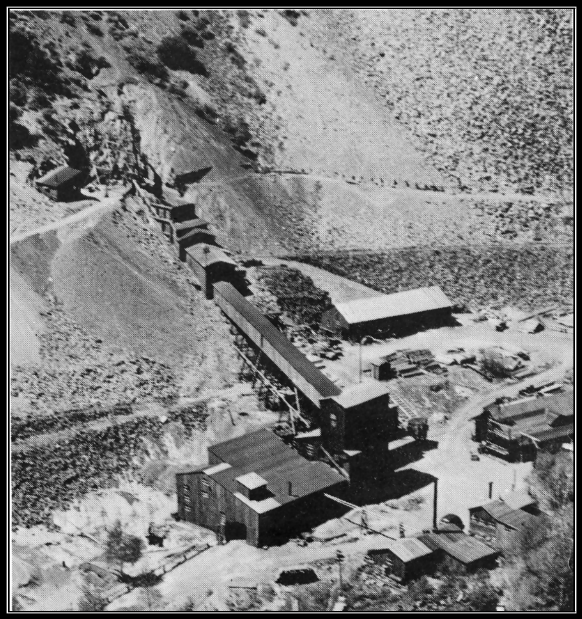
Figure 16. Aerial view of the Clayton Silver Mines' mill and surface plant, May 1939 (Clayton Silver Mines, Inc., The Golden Anniversary).
