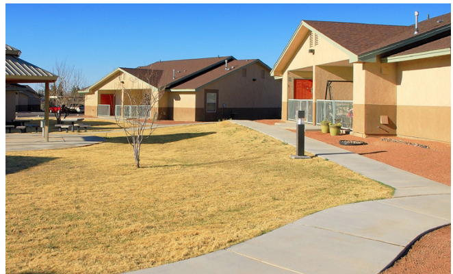
Mariposa Village Apartments.
