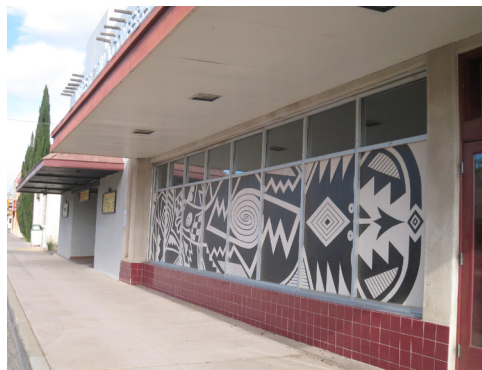
Painted storefront windows on Pine Street.
