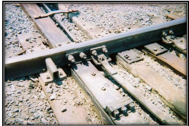
The second turnout at M.P. 1 is 115 lb composition that transitions down to 90 lb. rail. The switch point needs some repair; nine (9) switch ties need to be replaced.
