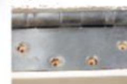
Figure 5 Completed hinge installation
