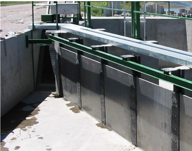
Staff constructed this solar powered, vertical panel screen with wiper brush and belt screen cleaner on Simonsen #1 POD. The solar-powered belt screen transfers debris back into the water behind the screen.
