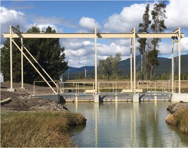
Pump Ditch, 26.9 cfs on the Wood River built by Central Point screens shop staff
