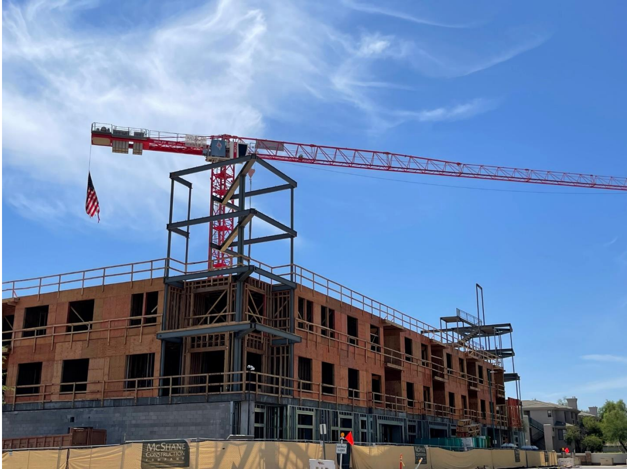
Figure 1: 1+5 Under construction, Scottsdale, AZ, 2021 (Kathy Howard) 15
