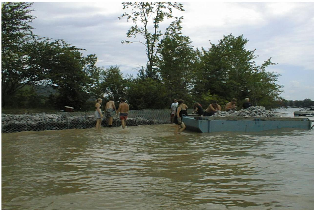
Hand carrying stone from the barge to the gabions due to lake being down.
