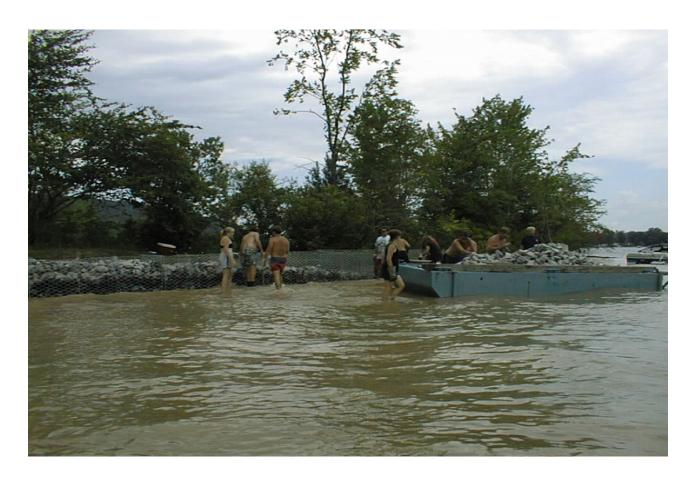
Hand carrying stone from the barge to the gabions due to lake being down.
