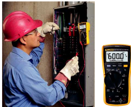
Figure 1-11 Testing for the presence of voltage. Photos courtesy Fluke, www.fluke.com . Reproduced with Permission.
