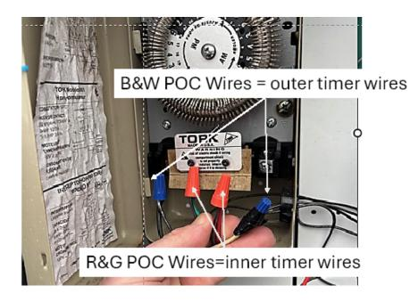
Tip: If you have an existing timer, the two outer wires going into timer are power wires, and the inner wires are control wires. Just remove wires from timer and wire into POC.
