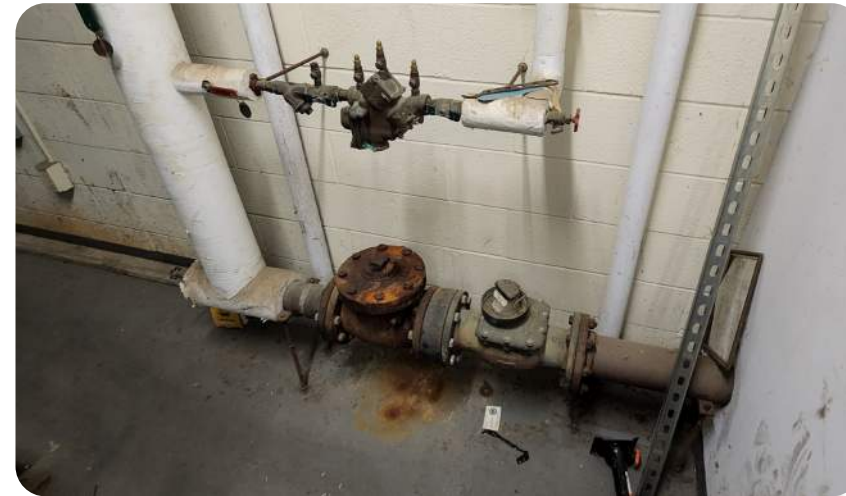
Water service in poor condition
