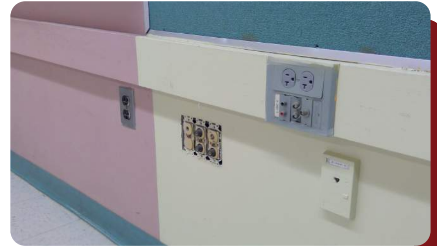
All surface-mounted electrical/data
