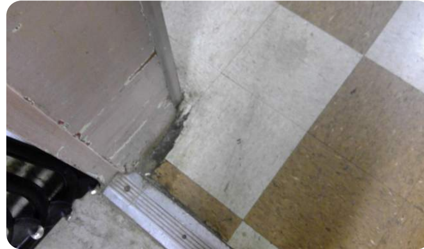
Cafeteria flooring general wear
