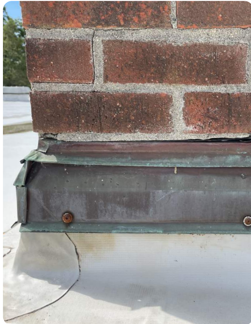
Cracked, settling brick compromising existing flashing
