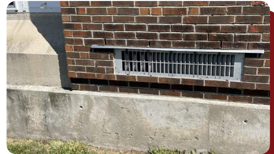
Damaged grille for unit ventilator, typ.
