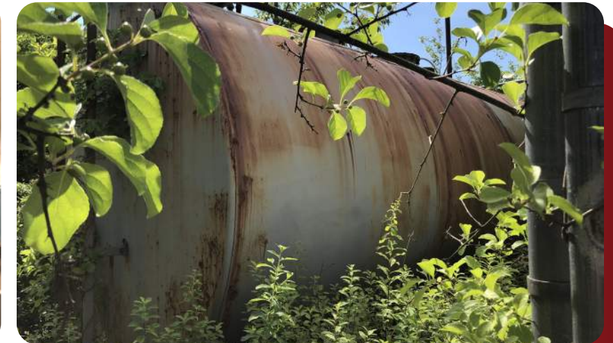
Abandoned fuel oil storage tank
