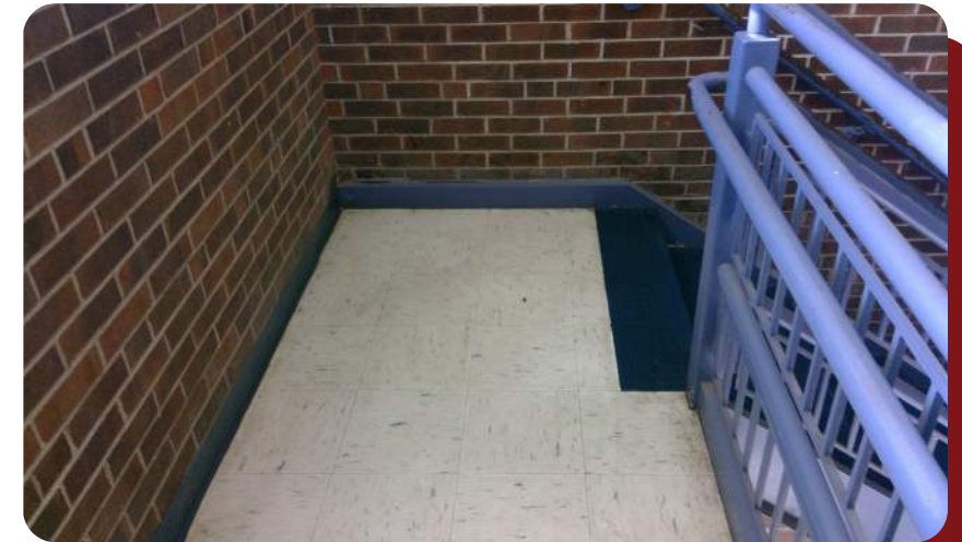
Narrow egress stairs and landings
