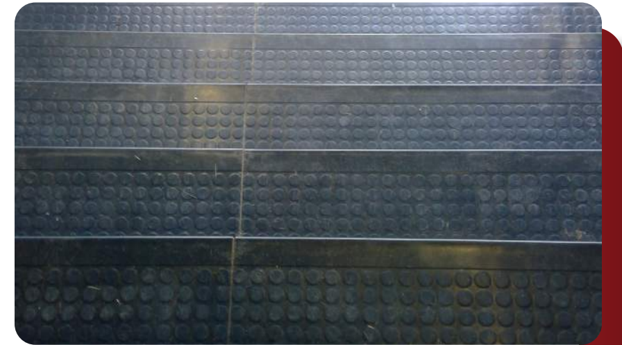
No visual impairment strips on stairs
