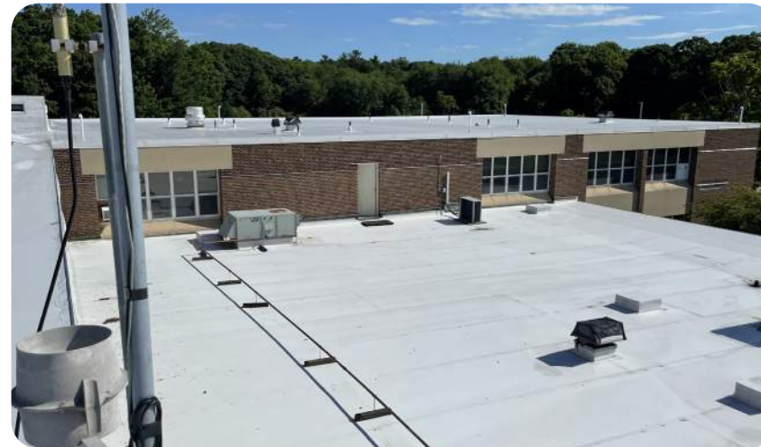
Non-compliant exterior walls; heat gain occurring at existing classrooms
