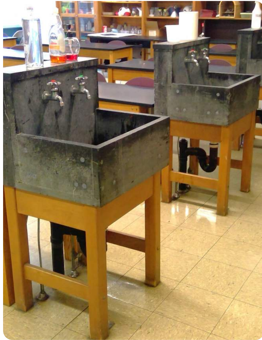
Existing, non-compliant, freestanding epoxy sinks in science classrooms
