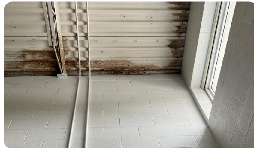
Water infiltration and rust at underside of roof deck (turf gym)
