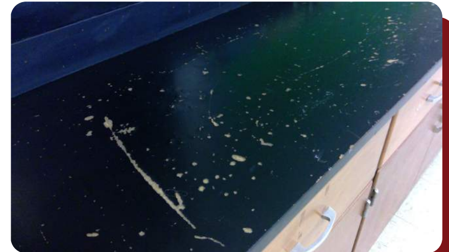
Typical science classroom countertop
