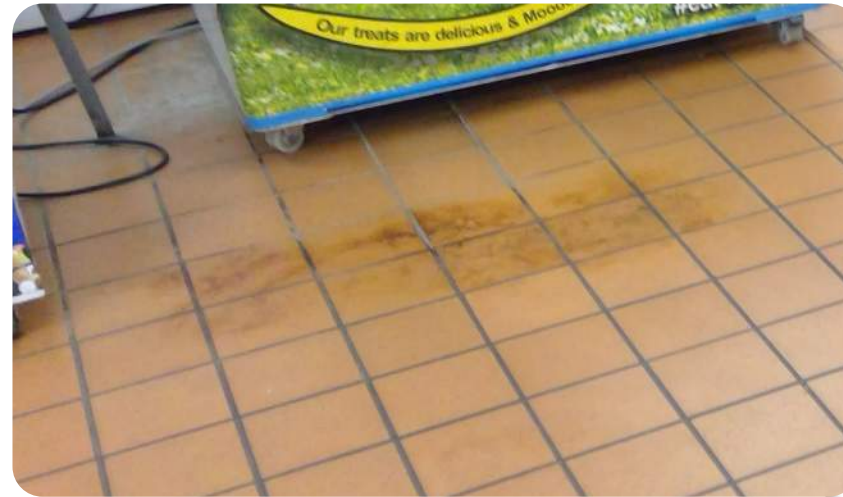
Stained kitchen quarry tiles
