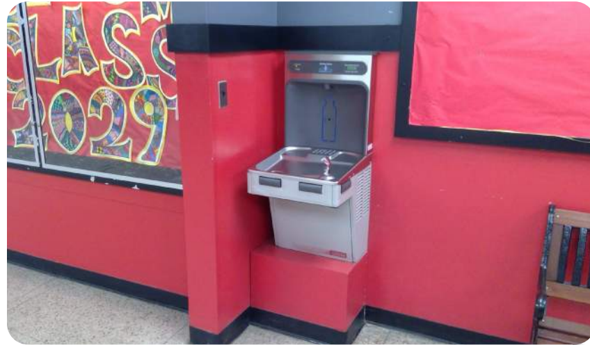
Lack of ADA accessible amenities
