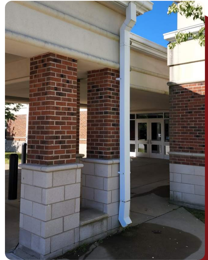
Downspout discharging at grade
