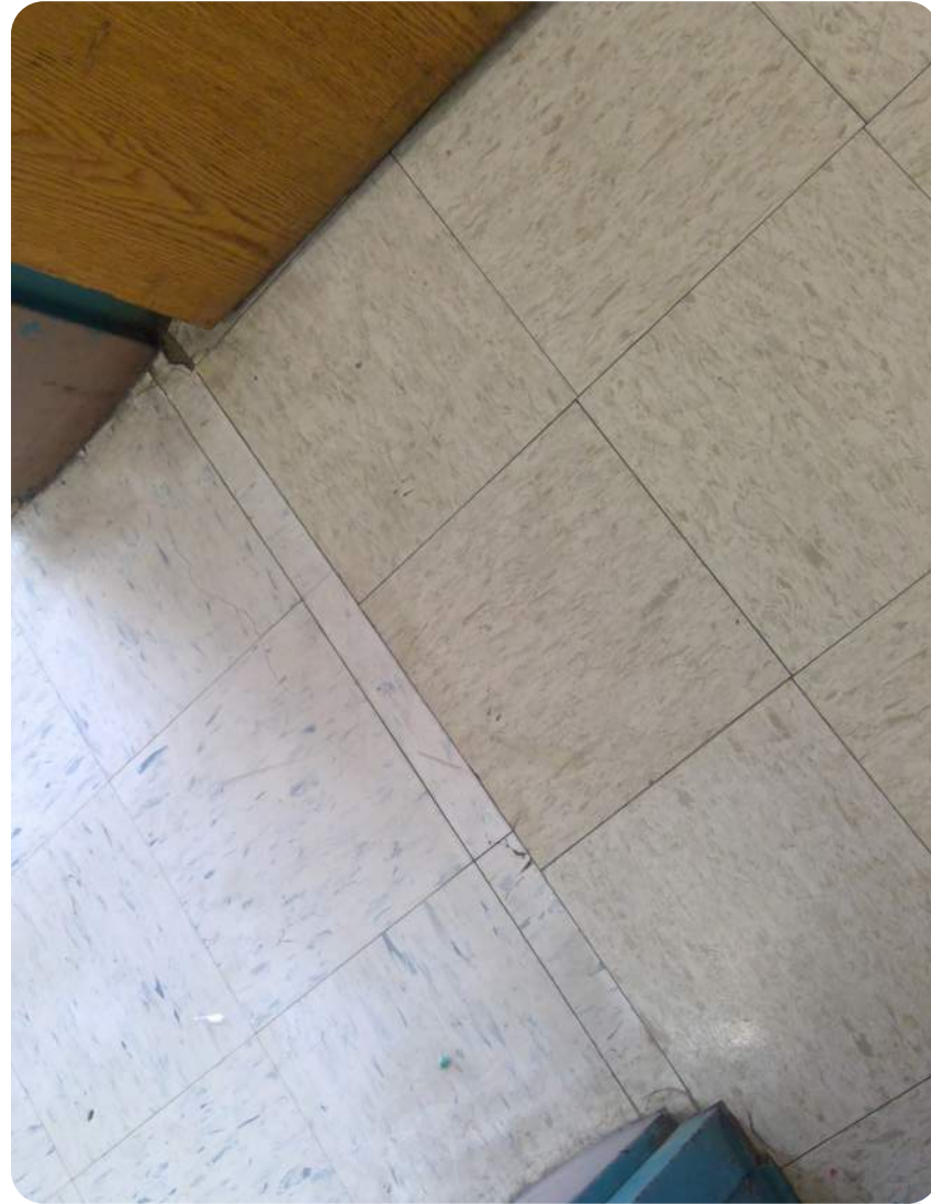
Typical condition of classroom flooring
