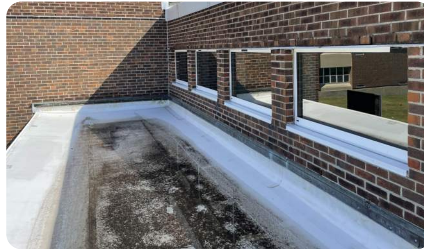
Water ponding - lack of proper drainage
