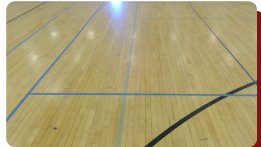
Gym flooring; includes warping, cupping, gaps & dead spots
