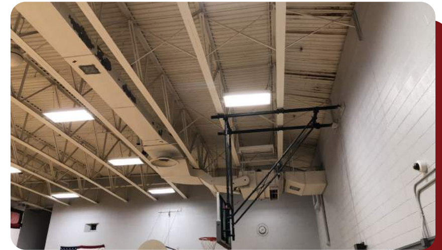
Gym indoor AHU's - outlived service life
