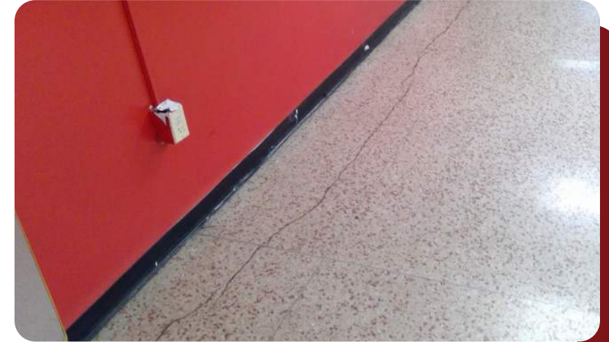
Epoxy terrazzo floors cracking
