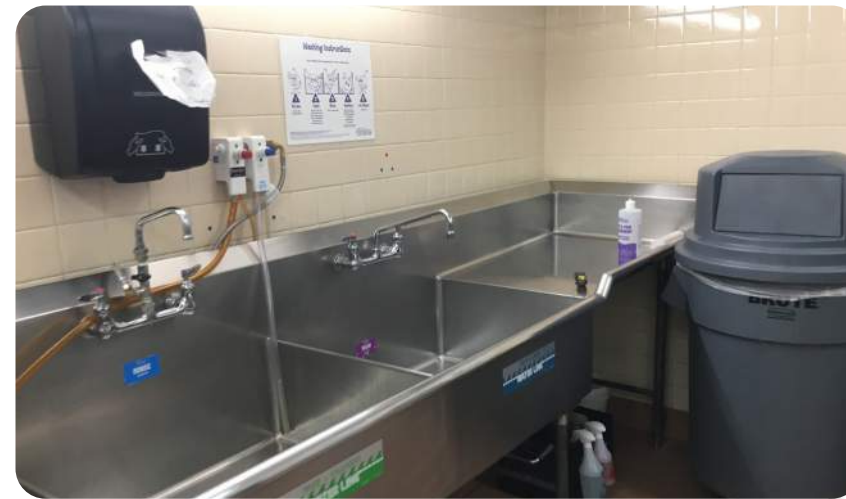
No grease interceptor at kitchen sinks
