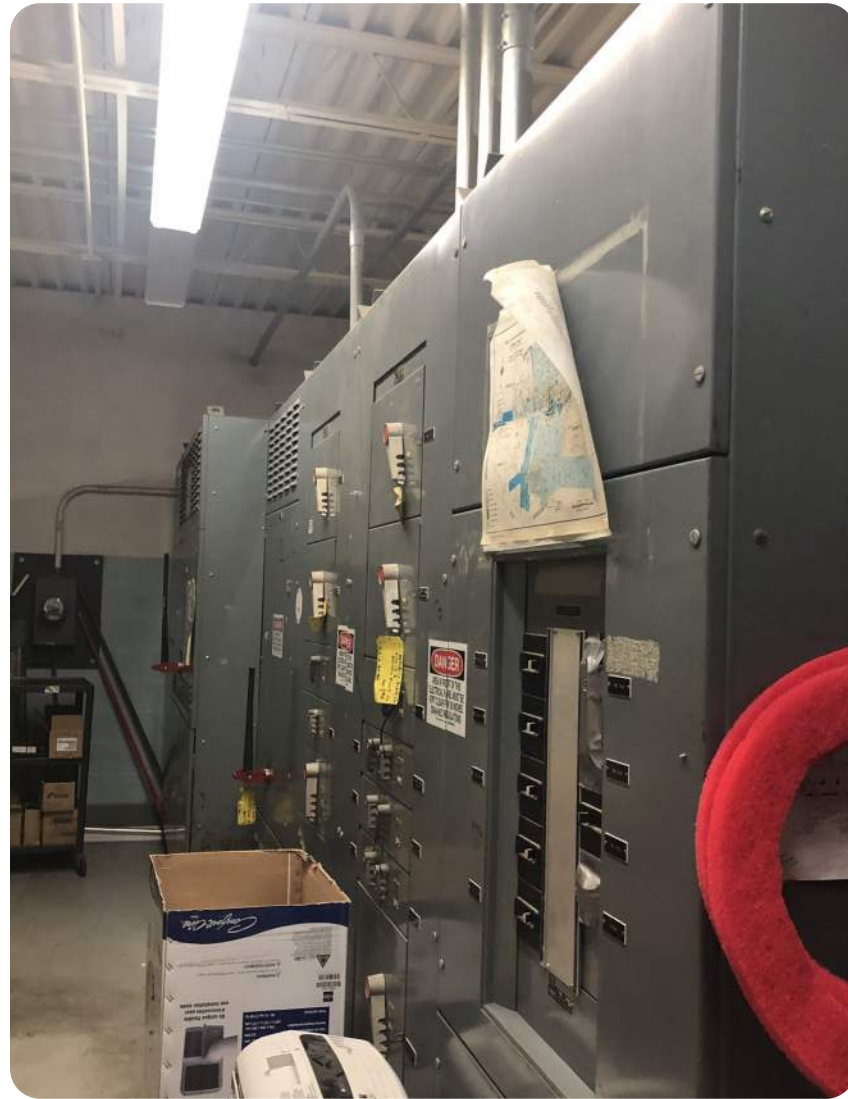
Normal power system in poor condition
