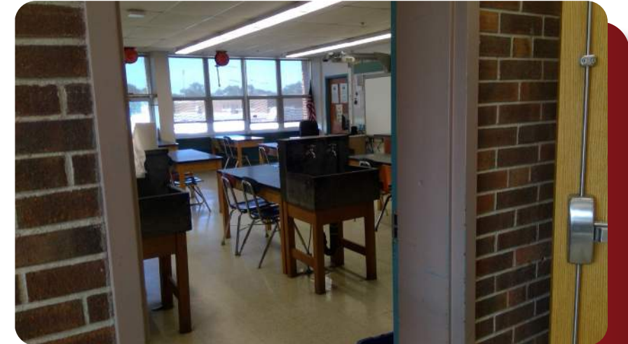
Door frame recesses too deep
