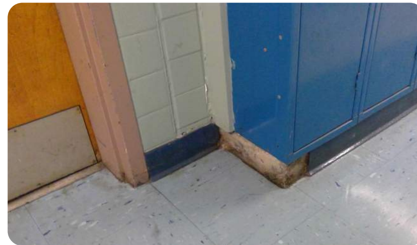
Missing finishes and general wear
