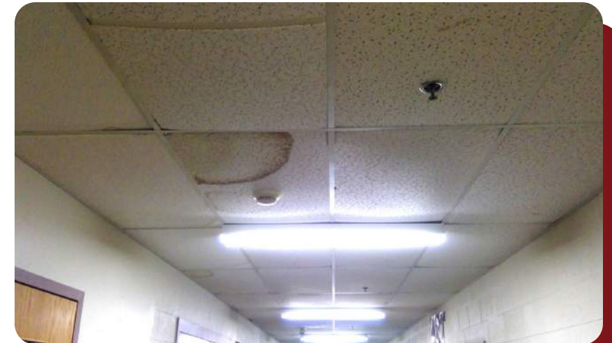
Sagging and stained corridor ceilings
