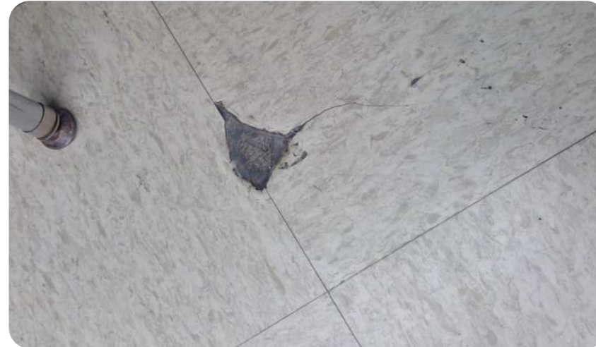
Typical condition of classroom flooring
