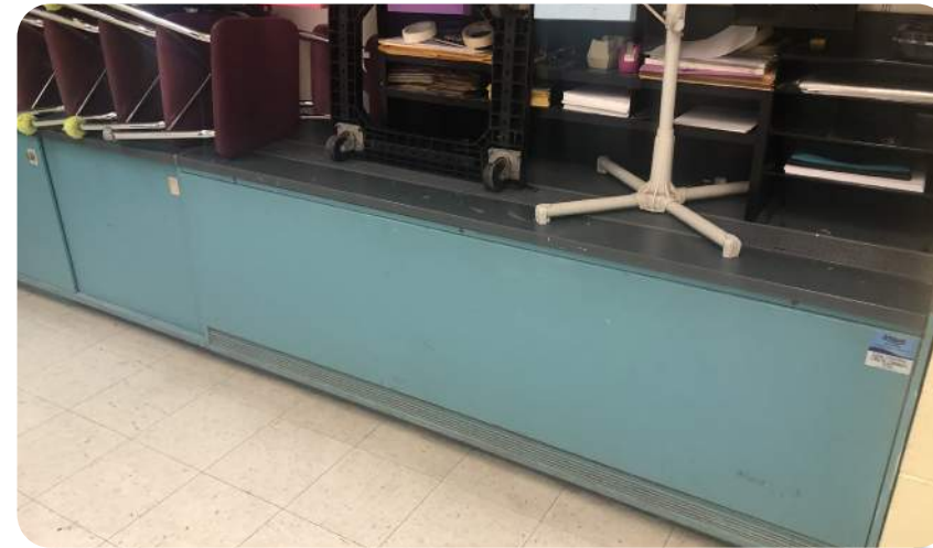
Unit ventilators; issues with uneven heating, ventilation, and acoustics
