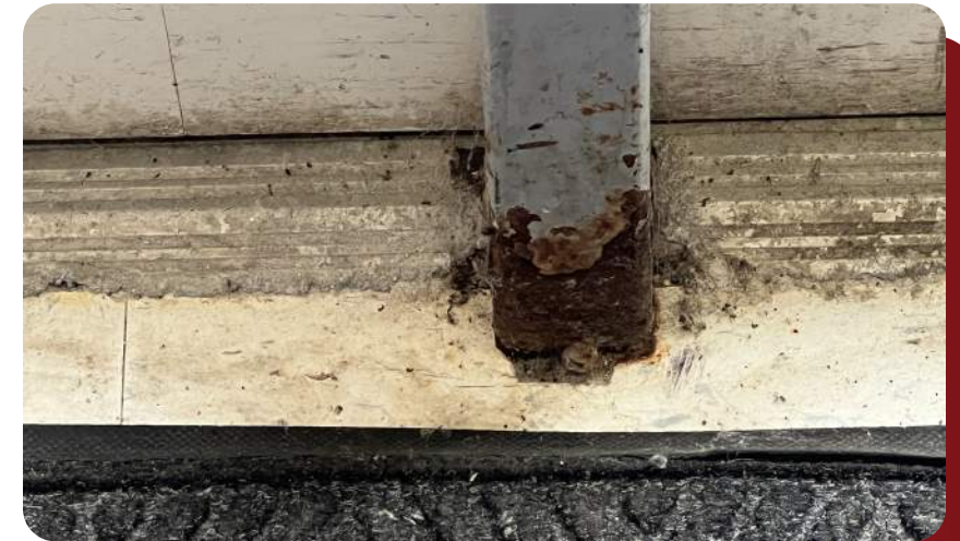
Rusting at exterior door frames
