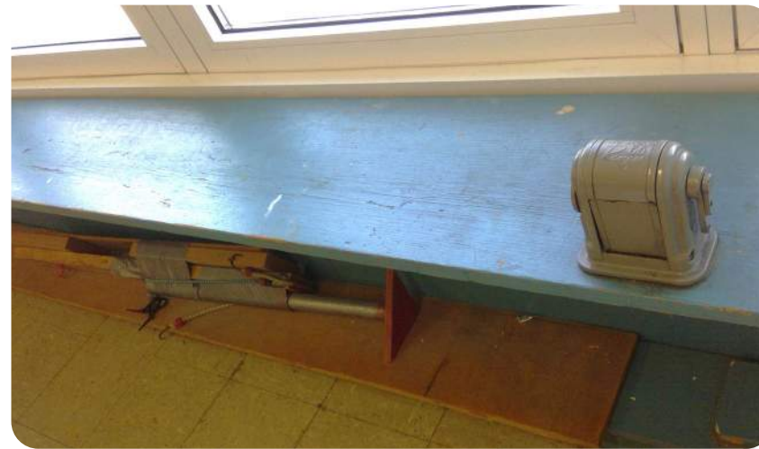
No classroom casework, chipped sills
