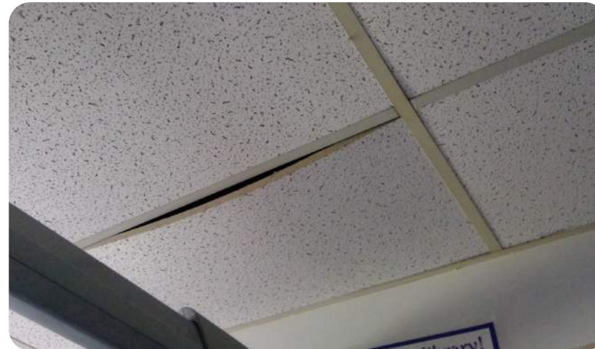
Discolored ceiling grids, typical
