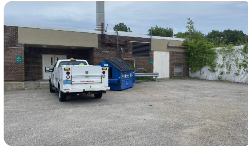
Existing loading dock area
