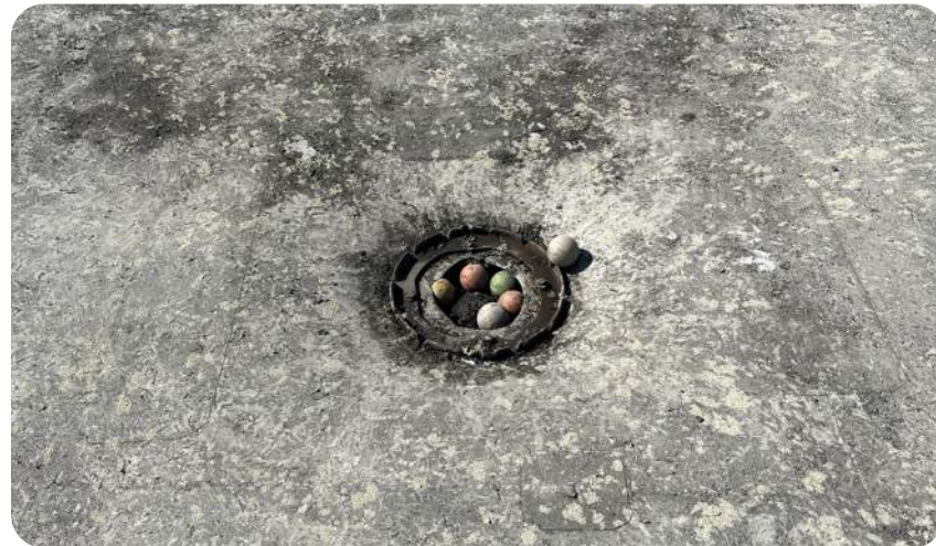
Roof drain strainers missing and roof membrane at end of useful life
