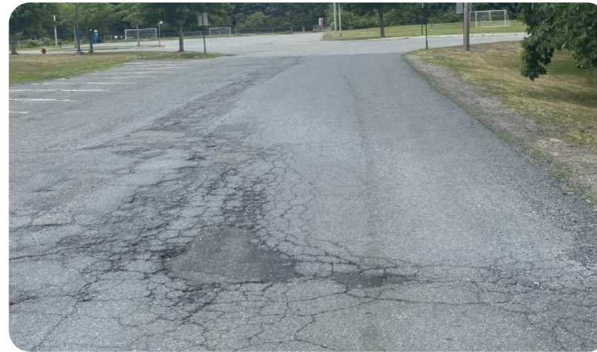
Deteriorated asphalt pavement with no curbing
