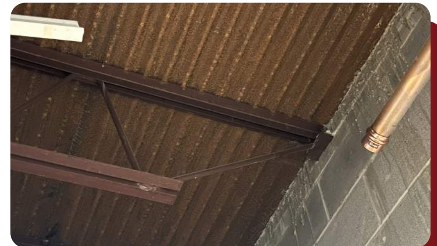
Rust at bottom of second floor deck with a history of mold issues
