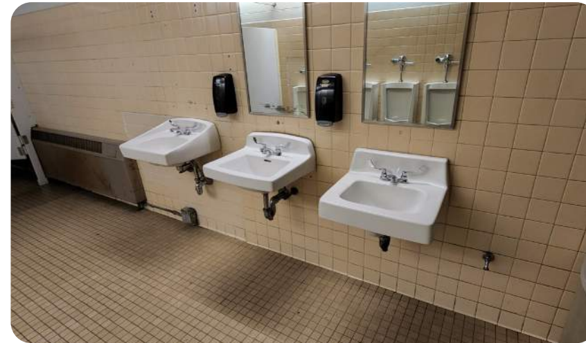
Lack of ADA accessible sinks
