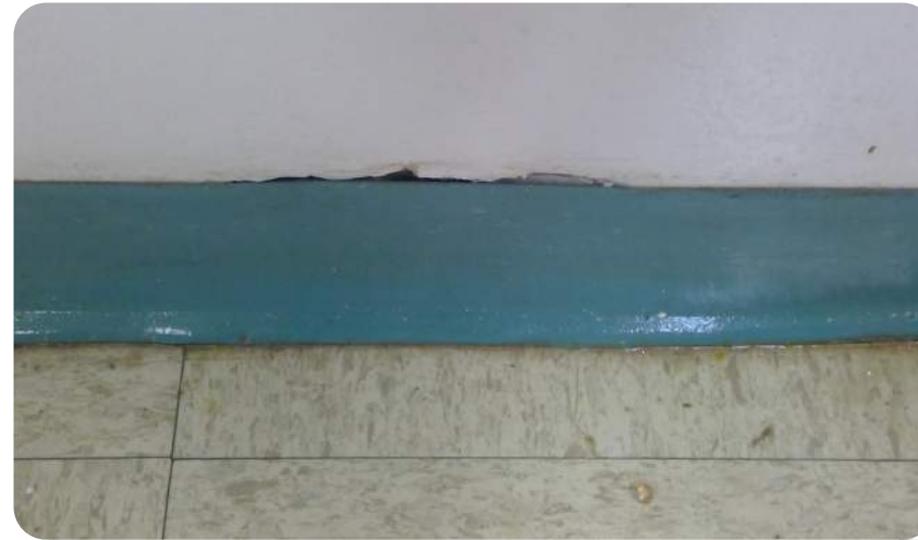
Rubber base with no wall behind
