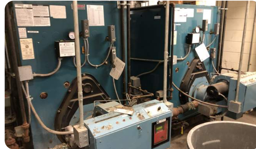
Boilers past useful service life
