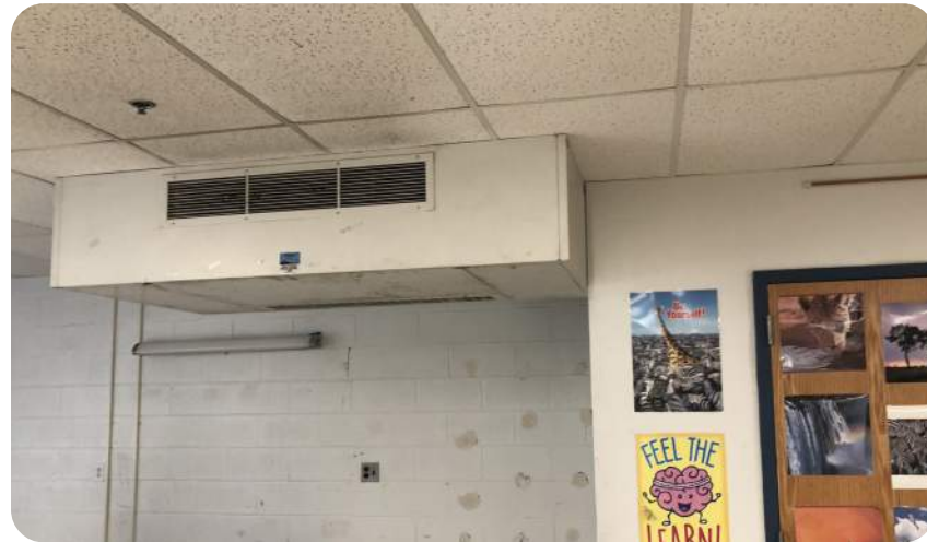
Ductless units reduce ceiling heights
