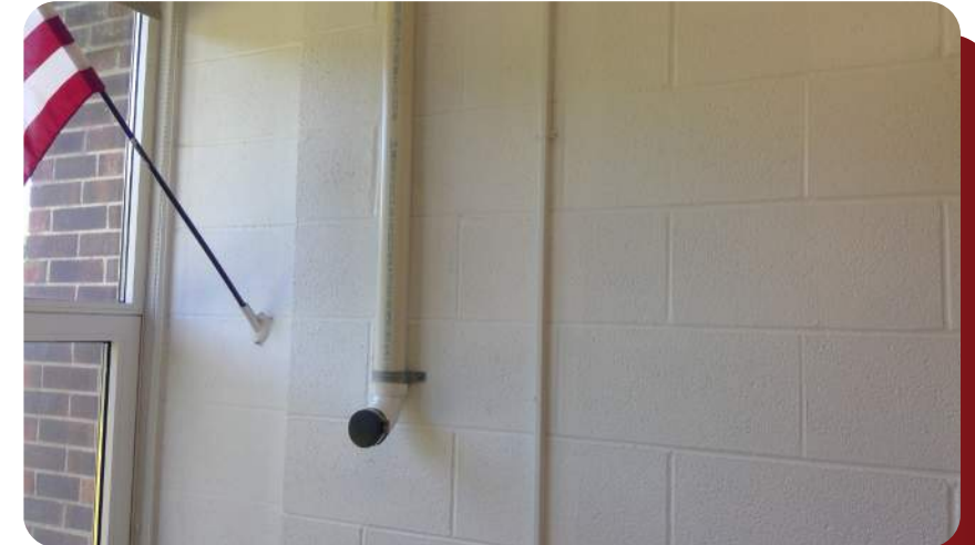
Typical example of exposed piping
