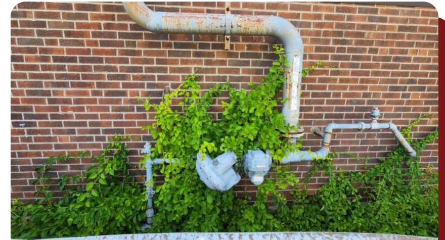
Gas system in fair condition
