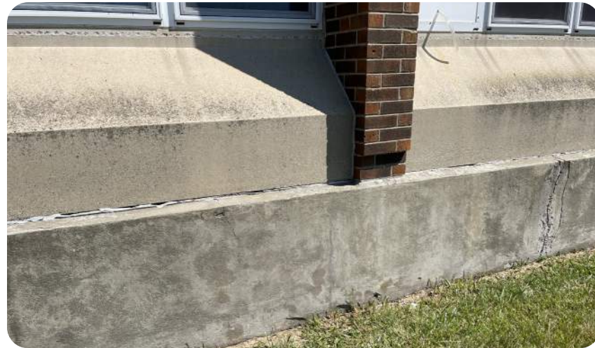
Spalling of exterior concrete foundations
