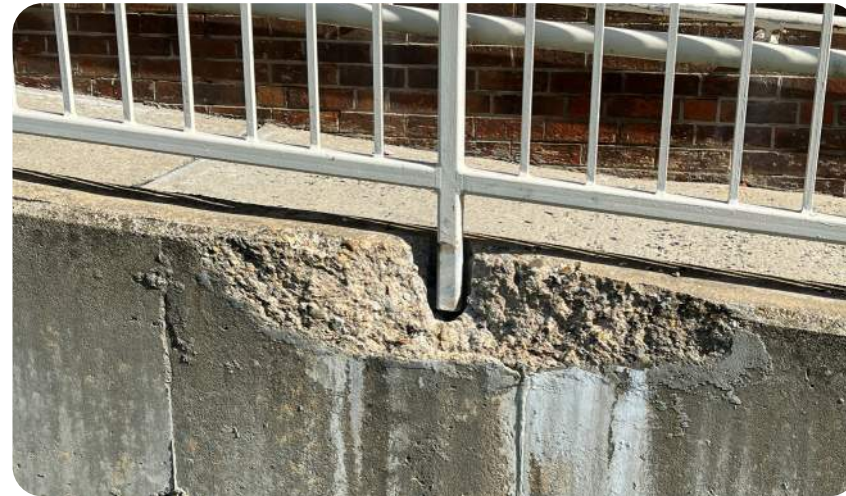
Damage at exterior ramp
