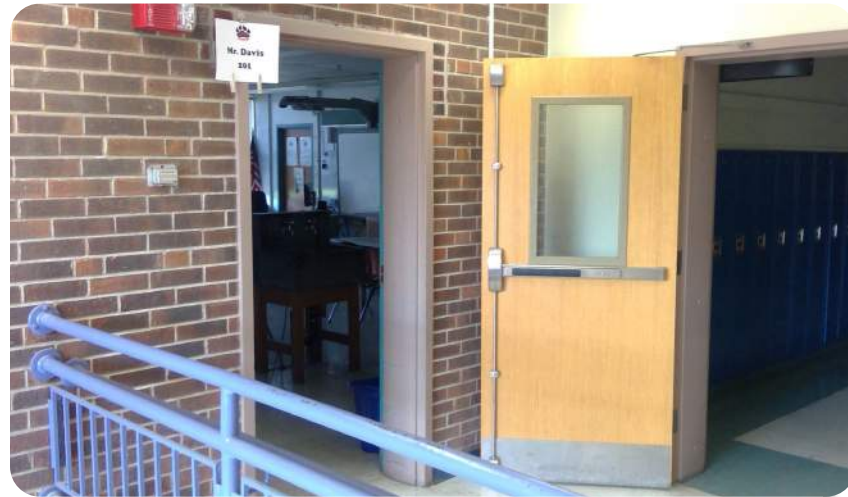
Classrooms only accessed from egress stairs - non-compliant
