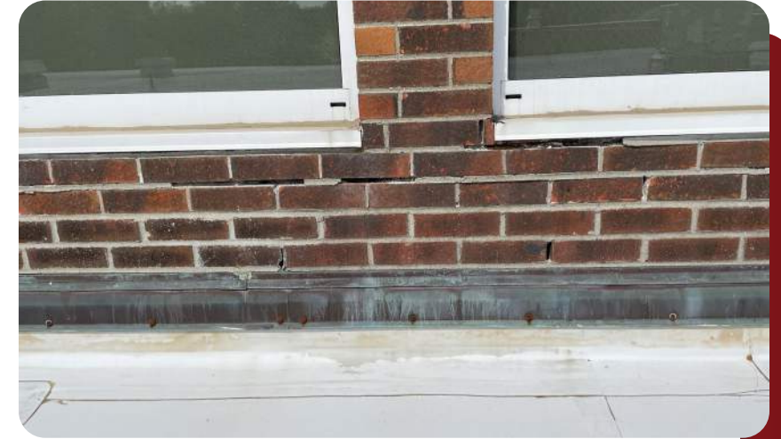
Water infiltration at exterior walls causing mortar joints to fail
