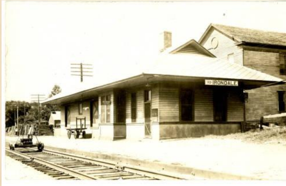
Irondale railroad station Mo, 1900s from SHSMO
